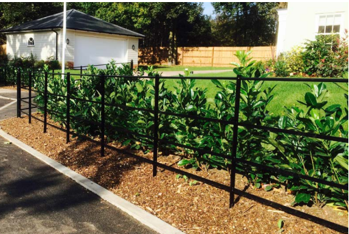
Metal estate railing in combination with hedging
