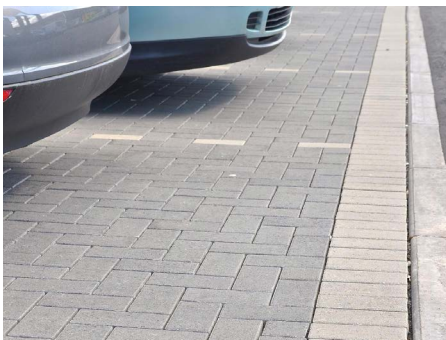
Block paving to vehicle parking bays
