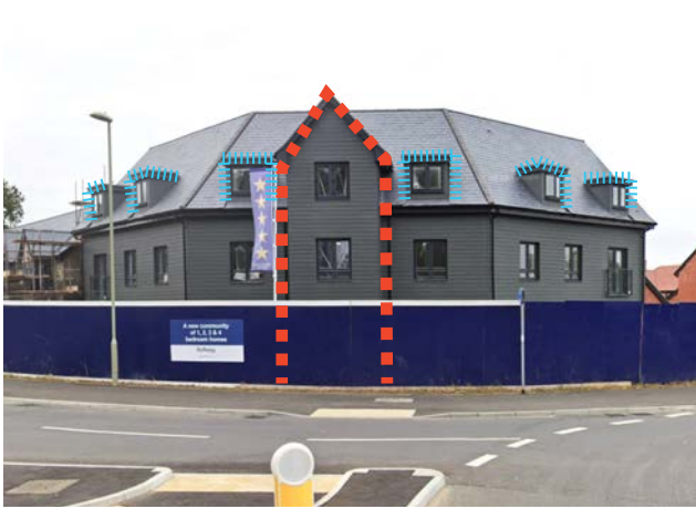
02 2.5 storey corner to new estate roundabout
