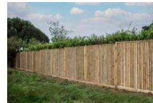
Timber closed board fence
