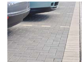
Block paving to vehicle parking bays
