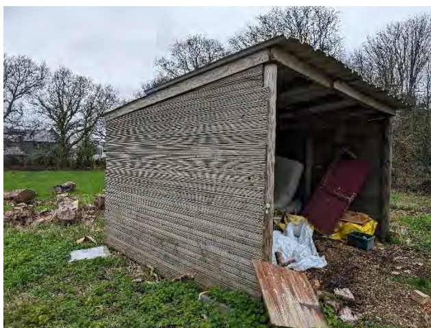
Photo 35. The southwestern elevation of building 7.
