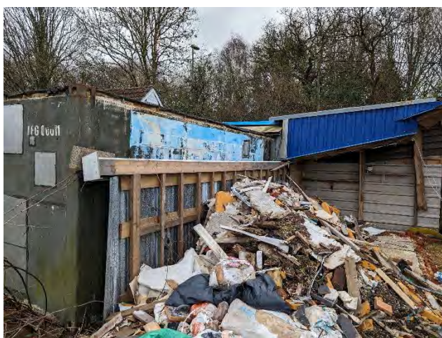
Photo 11. The southeastern elevation of building 2.
