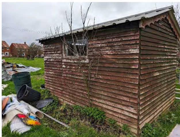
Photo 26. The southern elevation of building 5.
