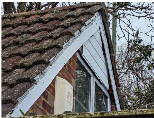
Photo 16. The southeastern gable end of building 3.
