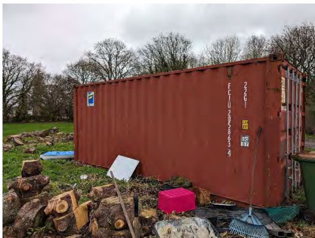
Photo 31. The southwestern elevation of building 6.
