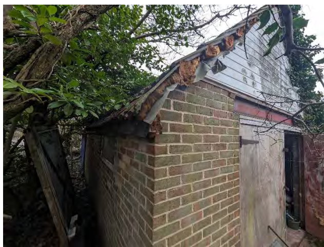
Photo 15. The northeastern elevation of building 3.
