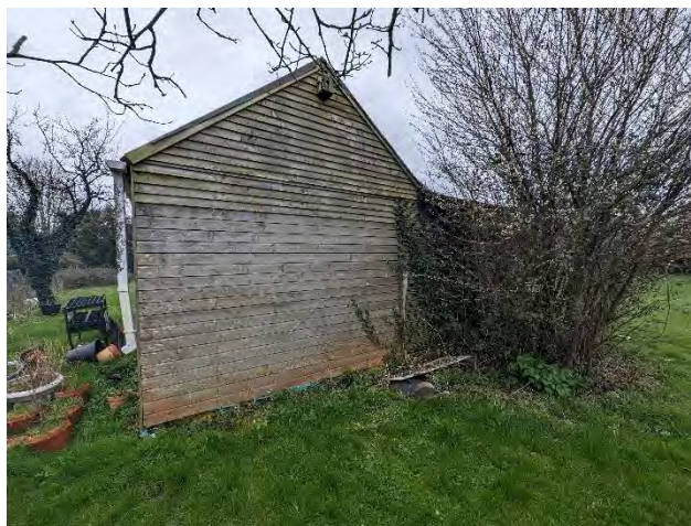
Photo 38. The northern elevation of building 8.
