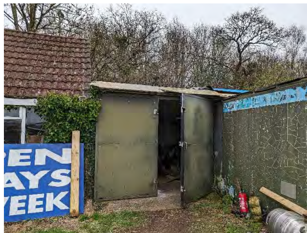
Photo 8. The southwestern elevation of building 1.
