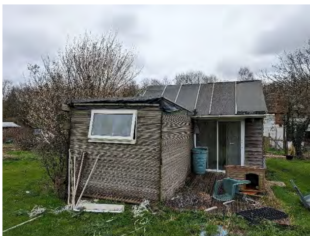
Photo 41. The western elevation of building 8.
