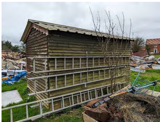
Photo 24. The northern elevation of building 5.
