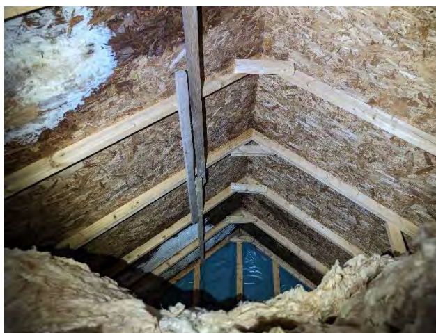
Photo 42. The internal area of the roof void of section a of building 8.
