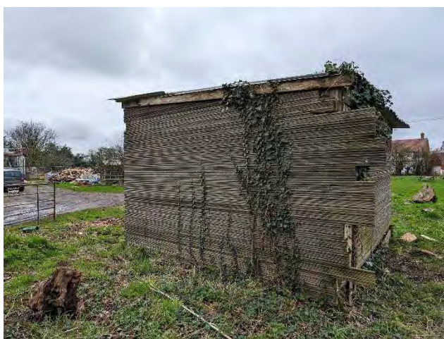
Photo 33. The northeastern elevation of building 7.
