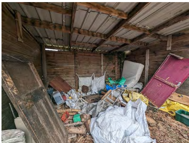
Photo 37. The internal area of building 7.
