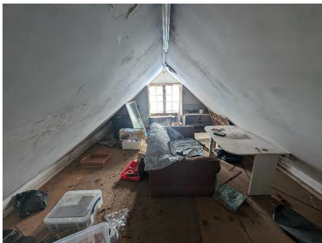
Photo 19. The internal area of the roof void of building 3.
