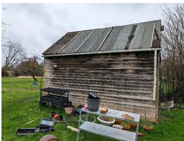
Photo 39. The eastern elevation of building 8.
