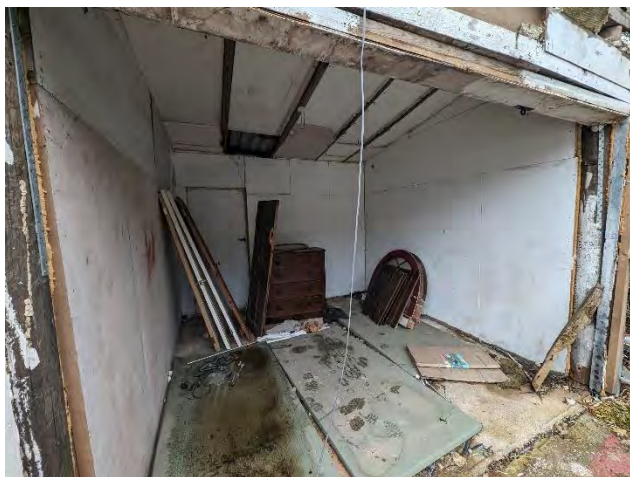
Photo 23. The internal area of building 4.
