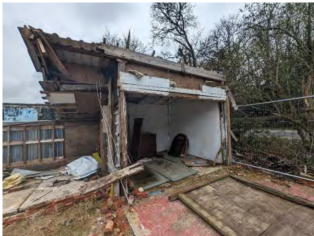
Photo 21. The southeastern elevation of building 4.
