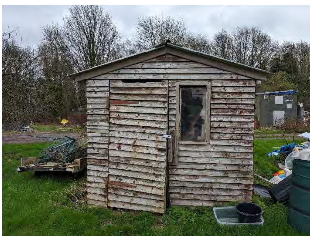
Photo 27. The western elevation of building 5.
