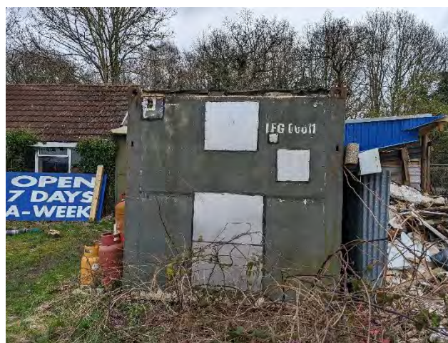
Photo 12. The southwestern elevation of building 2.
