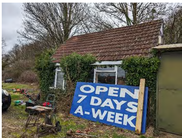
Photo 17. The southwestern elevation of building 3.
