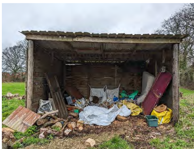
Photo 34. The southeastern elevation of building 7.
