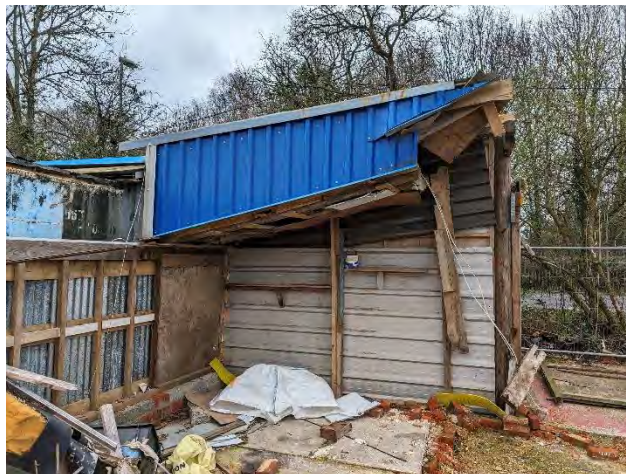
Photo 22. The southwestern elevation of building 4.
