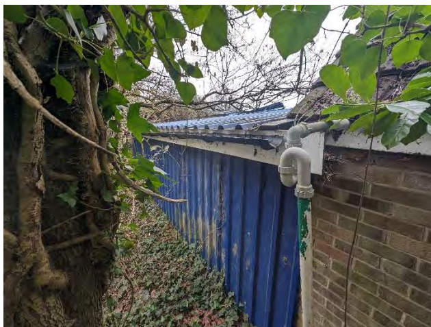
Photo 7. The northeastern elevation of building 1.
