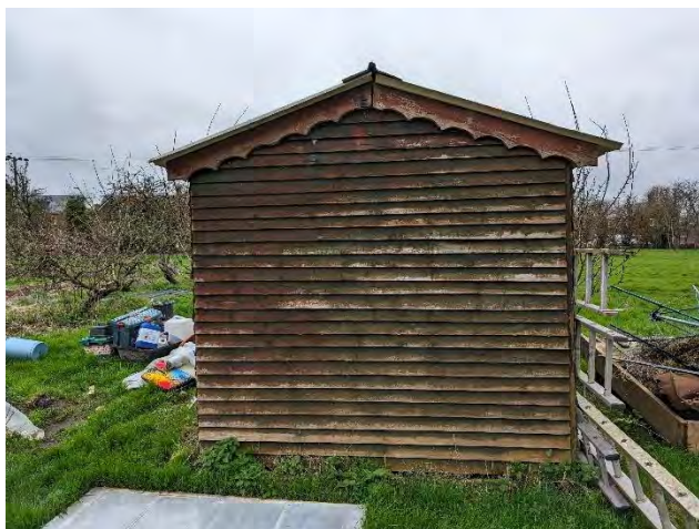
Photo 25. The eastern elevation of building 5.
