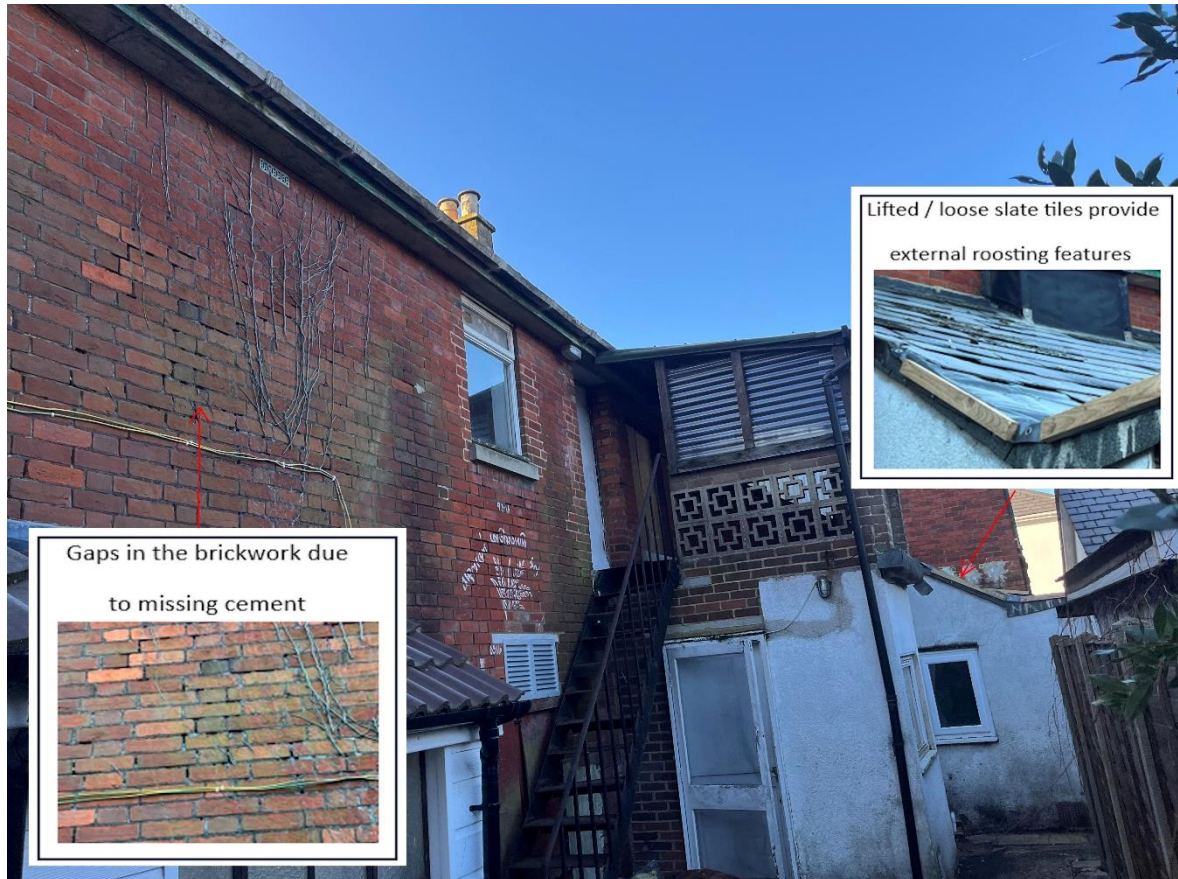
Image 4.3.1.1. Location of potential external roost locations on the north elevation of the building.
