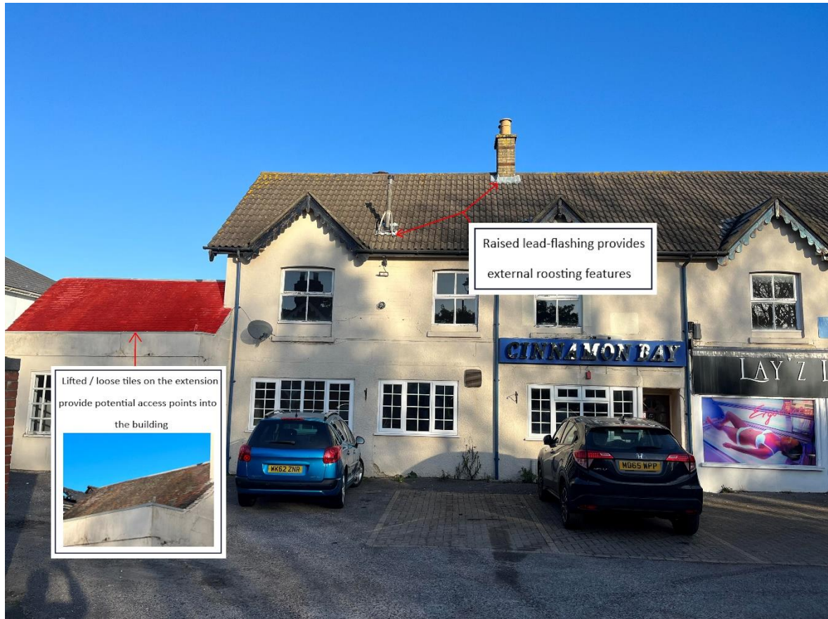
Image 4.3.1.2. Location of potential bat access points and potential external roost locations on the south elevation of the building.
