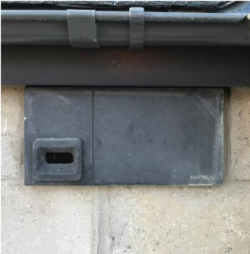
Figure 6. Showing an example of a integrated swift box.
