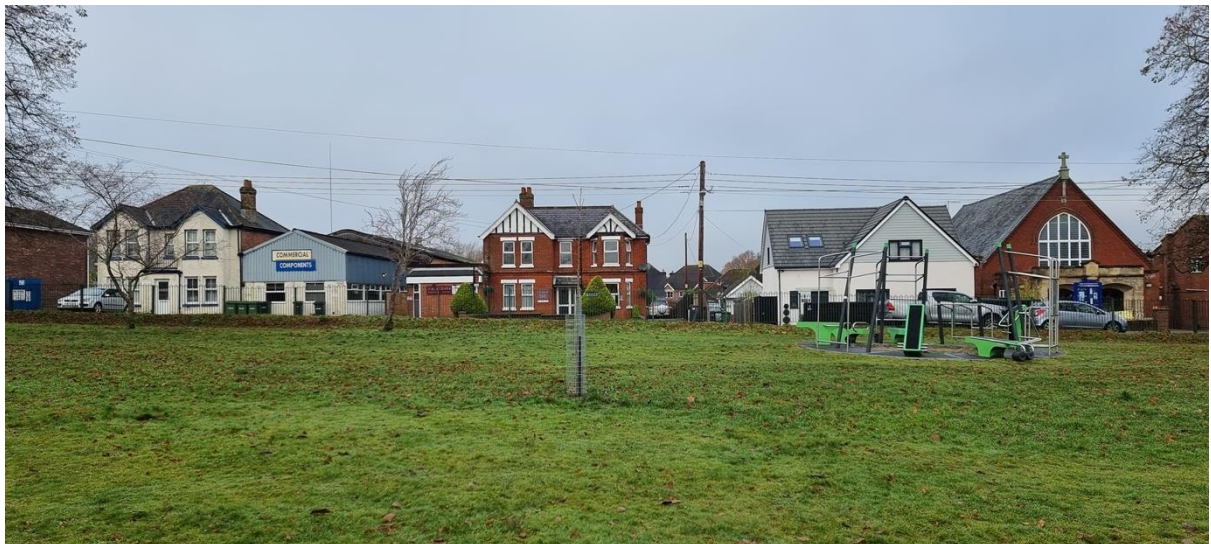
The above picture shows residential next to commercial and back land development at the same address, refer to aerial photo.
