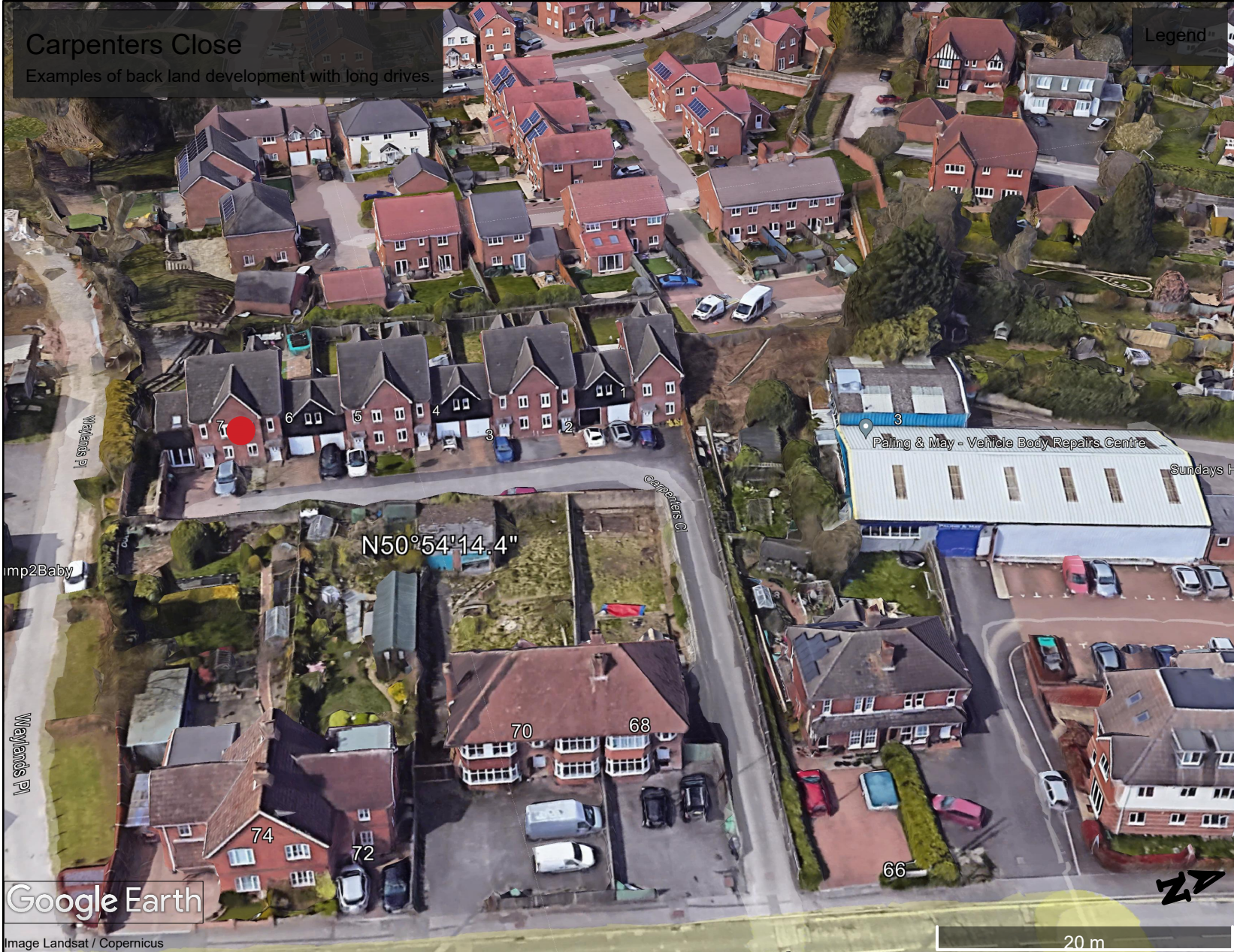
Carpenters Close - Hedge End - Shows no direct relationship with the street scene to allow for natural surveillance and neighbourly exchange. Development isolated from the street scene, and has a narrow drive with no visual connection with the street scene.
