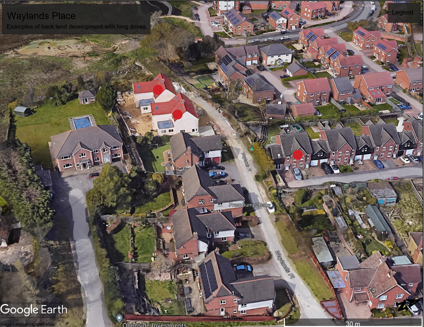
Waylands Place - Hedge End - Shows no direct relationship with the street scene to allow for natural surveillance and neighbourly exchange. Development isolated from the street scene.
