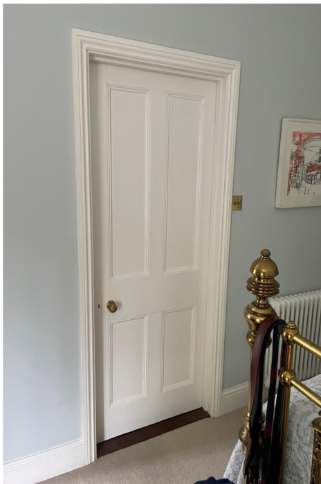
Remove door & make good wall. Reuse door into new dressing area.
