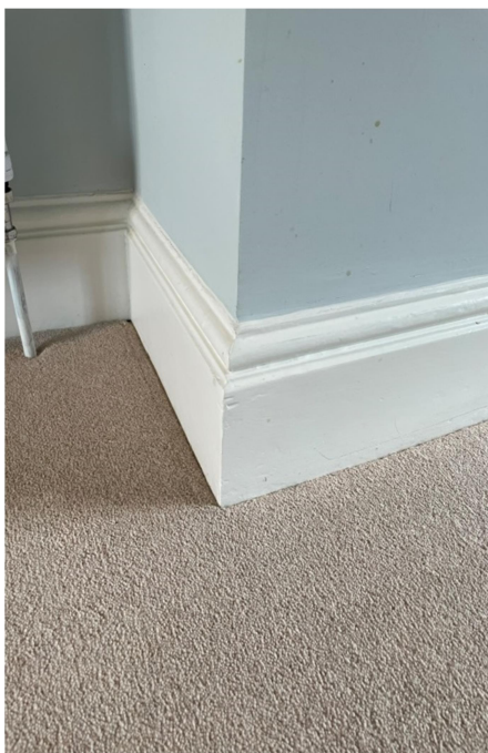
Remove & replace skirtings with deeper torus style to match main house
