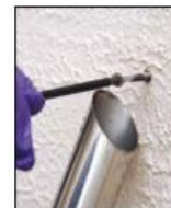
Control measures: shadow vacuuming and using a drill cowl as local extraction
