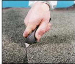
Cut and remove manageable sections
