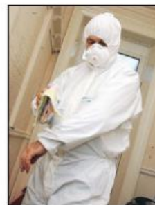
Cleaning with damp rag using patting action
