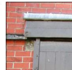
Built-up bituminous roofing and bituminous asbestos fabric over a doorway
