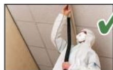
Disposable RPE worn correctly
