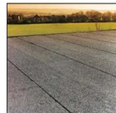
Built-up bituminous roofing and bituminous asbestos fabric over a doorway
