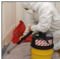
Vacuum clean carefully. It is easy to disturb asbestos fibres, make them airborne and breathe them in
