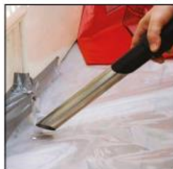
Vacuum clean carefully. It is easy to disturb asbestos fibres, make them airborne and breathe them in
