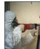
Control measures: shadow vacuuming and using a drill cowl as local extraction
