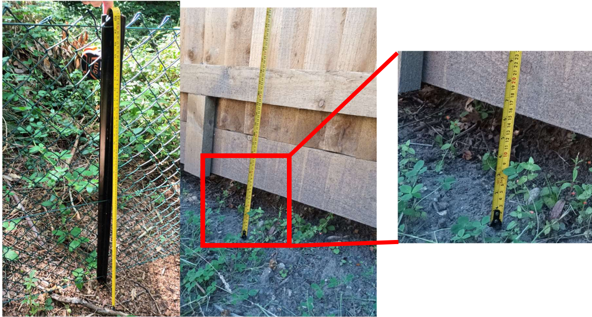
Figure 3 - Reduced height eco-friendly fencing installed – 150mm gaps introduced for wildlife under the fences
