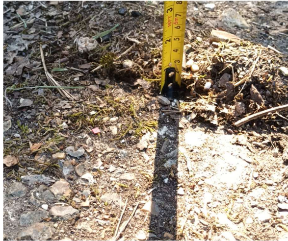
Figure 2 - 1950s concrete slab under the existing grass on top of the root protection area
