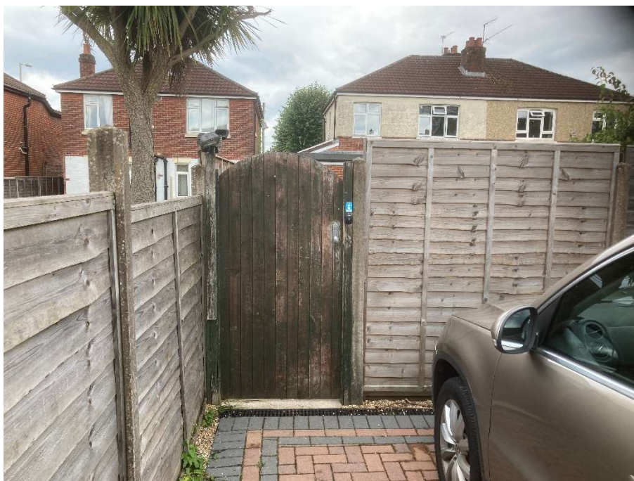
Fig. 7 – Photograph taken from the car parking area looking towards the high-level fence and security gate which provides access to the nursery and outdoor play area.
