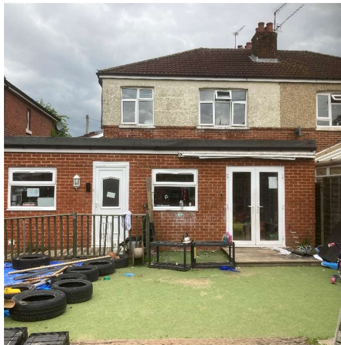
Fig.1 – Photograph taken from the outdoor play area looking towards the rear (south-west) elevation of the building at 177 Leigh Road
