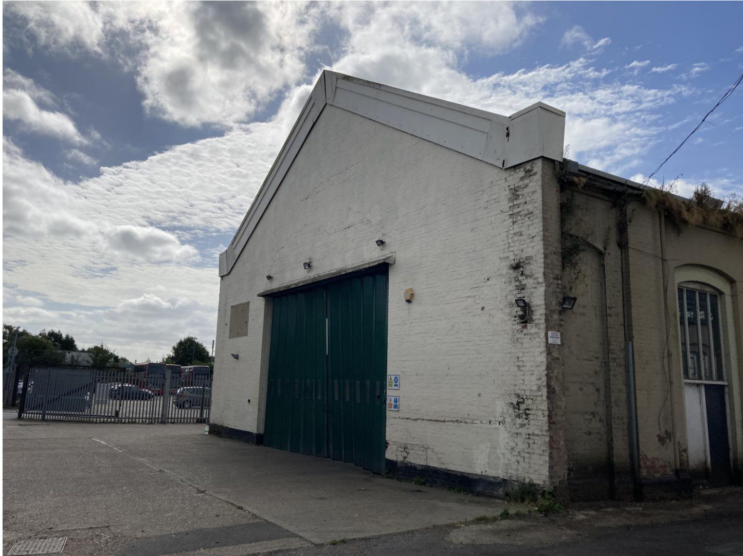
Figure 1 Existing North Elevation
