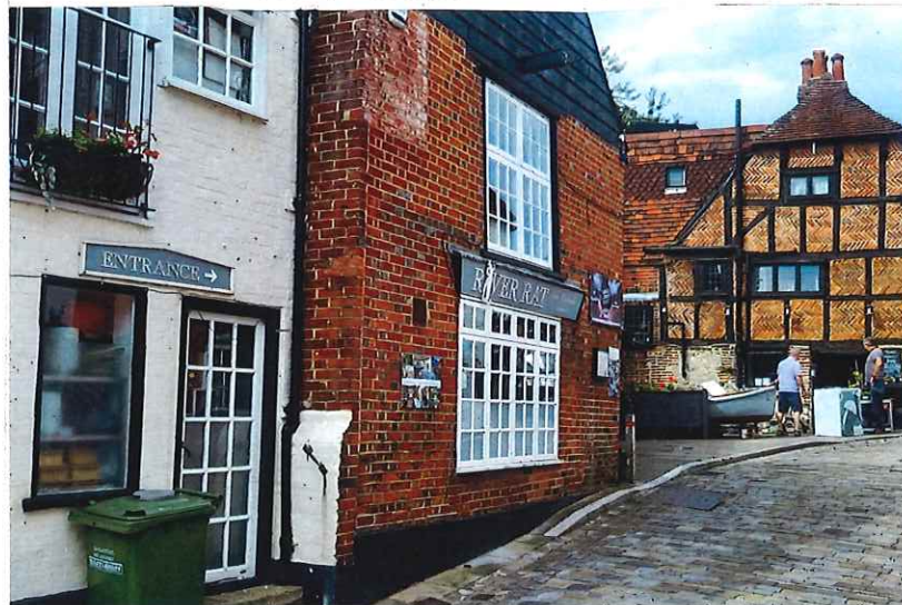
VIEW FROM HAMBLE HIGH STREET SHOWING MULTI PANE GLAZED DOOR TO KITCHEN, RIVER RAT RESTAURANT, AND OLD HOUSE IN THE BACKGROUND
