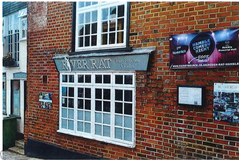
GROUND FLOOR WINDOW TO HIGH STREET OF RIVER RAT RESTAURANT
