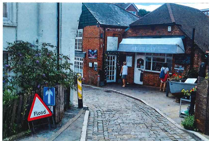
VIEW LOOKING DOWN HIGH STREET THROUGH NARROW OPENING SHOWING RIVER RAT RESTAURANT EXISTING DOORS AND CANOPY OVER FORECOURT
