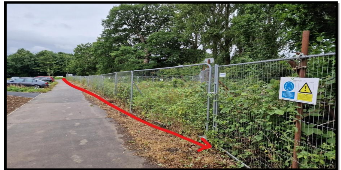
Image 17 – Red arrow indicates fencing to come down
