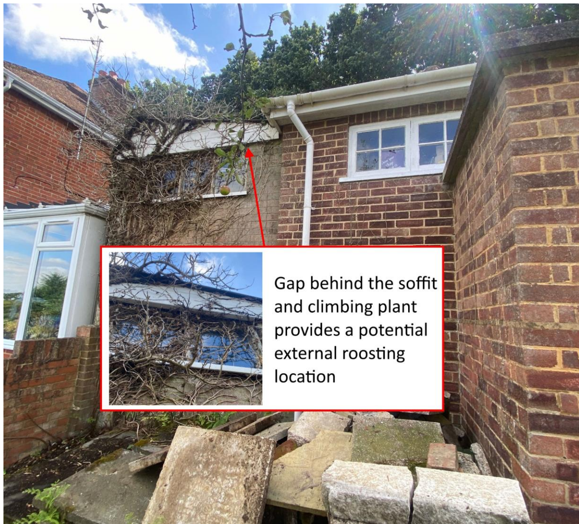
Image 4.3.2.1. Location of potential external roost location on the north-west elevation of the garage.
