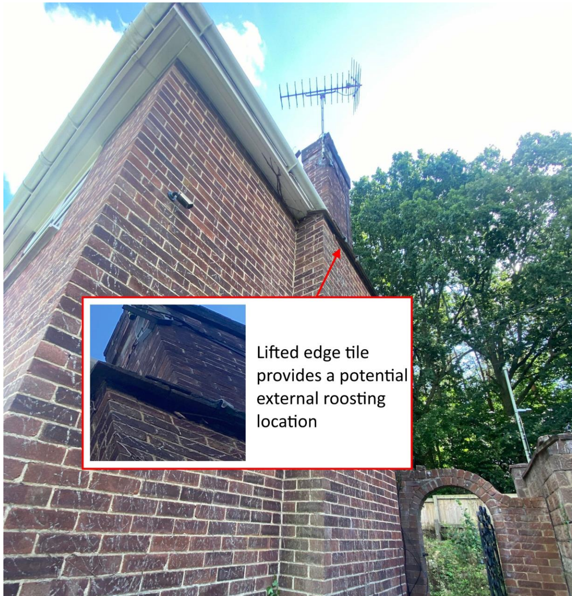
Image 4.3.1.1. Location of potential external roost location on the south-west elevation of the house.
