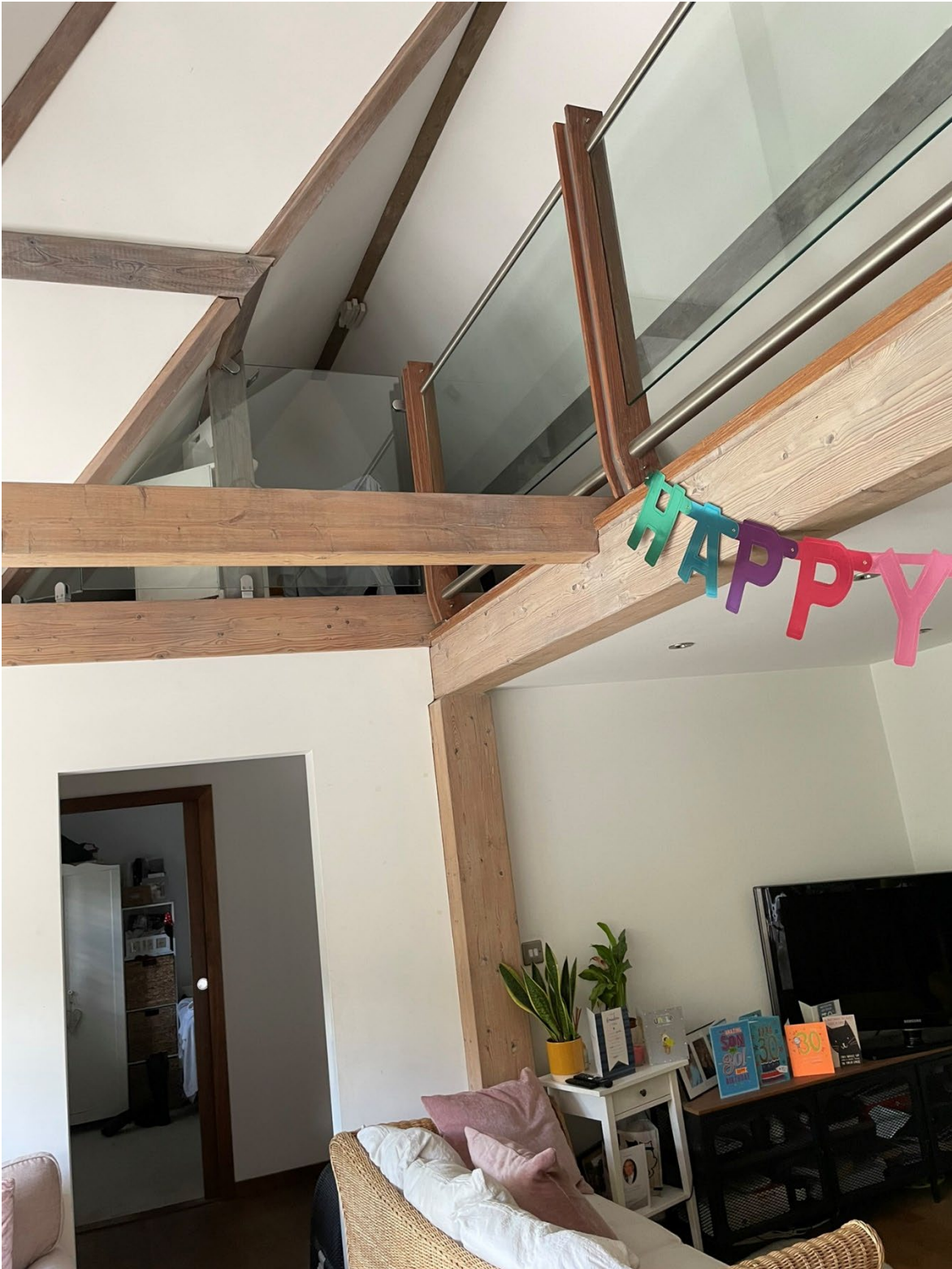
View of mezzanine gallery
