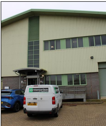
View of the front (east facing) elevation of the building
