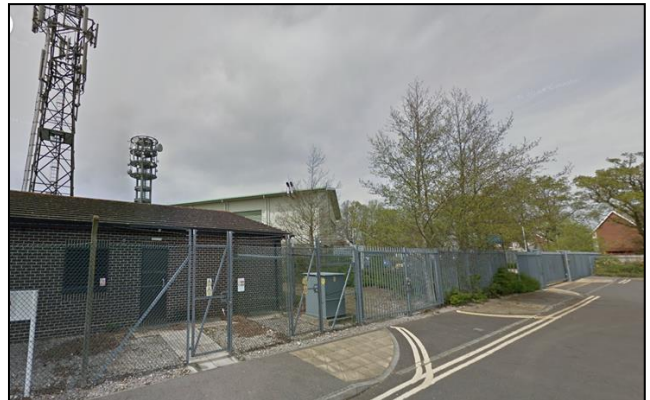
View showing the vehicular access to the site from Hamilton Way
