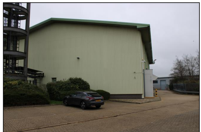
View of the west-facing elevation, also showing the base of the existing transmitter tower to be removed.
