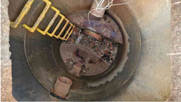
S24 (A)__TANK 5 (A)_7.jpg, 00:00:00, 0.00 m Start node, manhole, reference: S24 (A)
