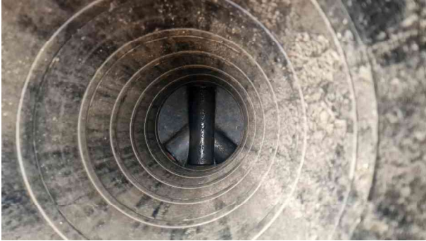
IC.1_DS_TANK 3_5.jpg, 00:00:00, 0.00 m Start node, inspection chamber, reference: IC.1
