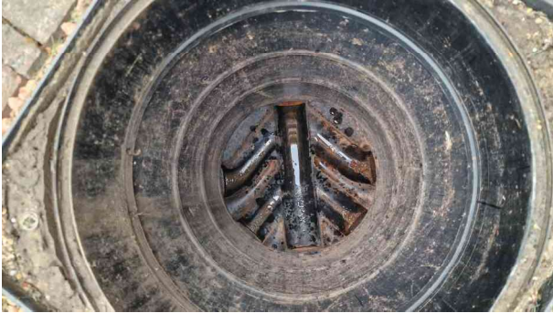
IC.2_DS_TANK 3_6.jpg, 00:00:00, 0.00 m Start node, inspection chamber, reference: IC.2
