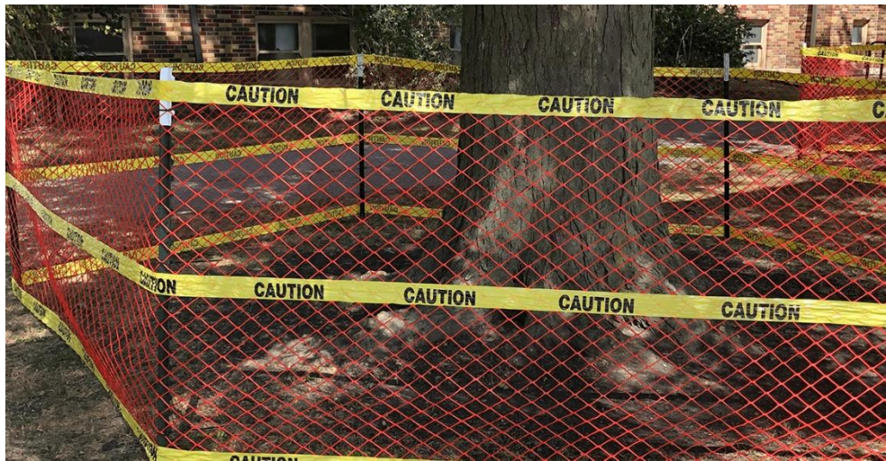
Figure 2: Tree stem protection example
