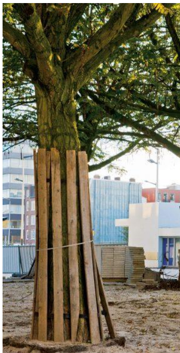
Figure 2: Tree stem protection example
