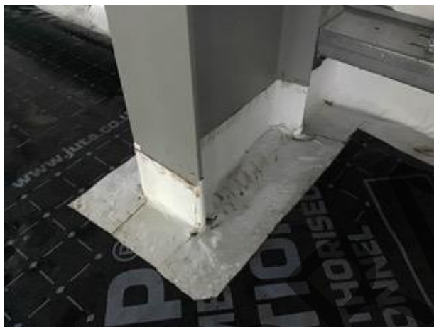
Typical stanchion seal using SAGM.
