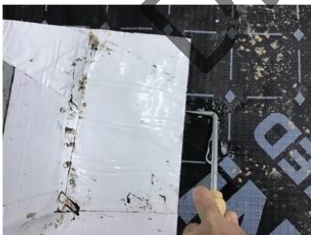
Pick testing all SAGM detailing.
