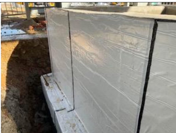
Unit 3/4. Juta GP SAM sealed continuously to lift pit wrap.
