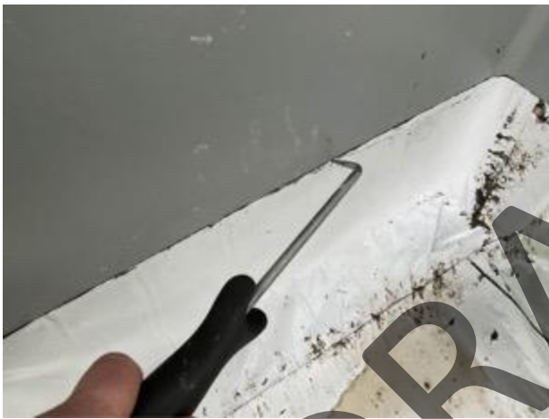
Pick test upon a sealed steel stanchion.
