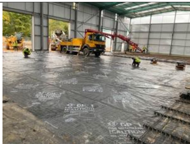
Overview of the installation of Juta GP1 Gas Barrier.
