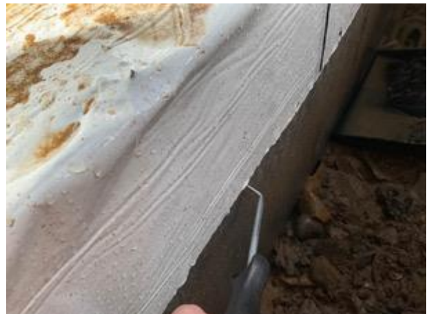
Unit 3/4. Pick test upon termination between membranes.
