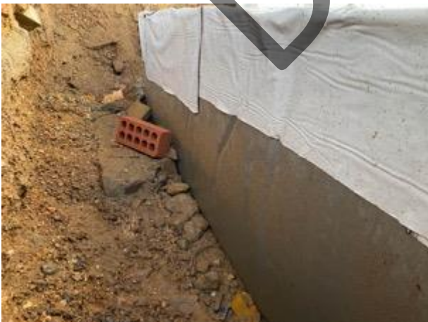
Unit 3/4. Juta GP SAM successfully terminated upon previously installed Juta TitanBond base.
