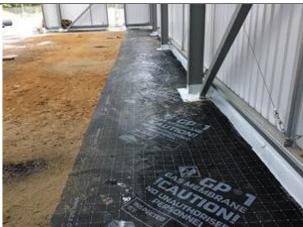
Overview of installed membrane to the perimeter of using 5.
