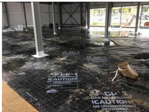
Overview of installed membrane under the mezzanine floor area.
