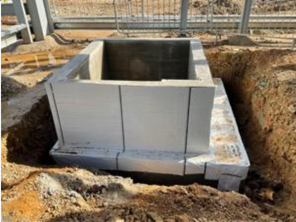
Unit 3/4. Overview of Lit pit wrap installation.
