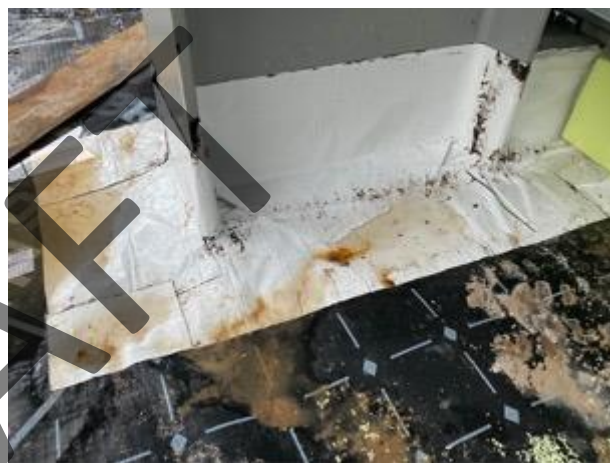
Typical steel stanchion sealed using SAGM
