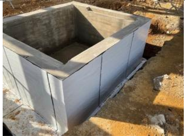
Unit 3/4. Overview of the installation of Juta GP SAM to lift pit.
