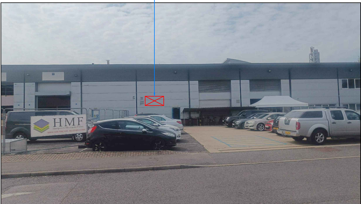
Existing Front Elevation Photo
