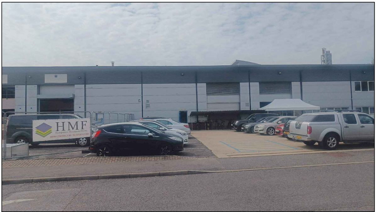
Existing Front Elevation Photo
