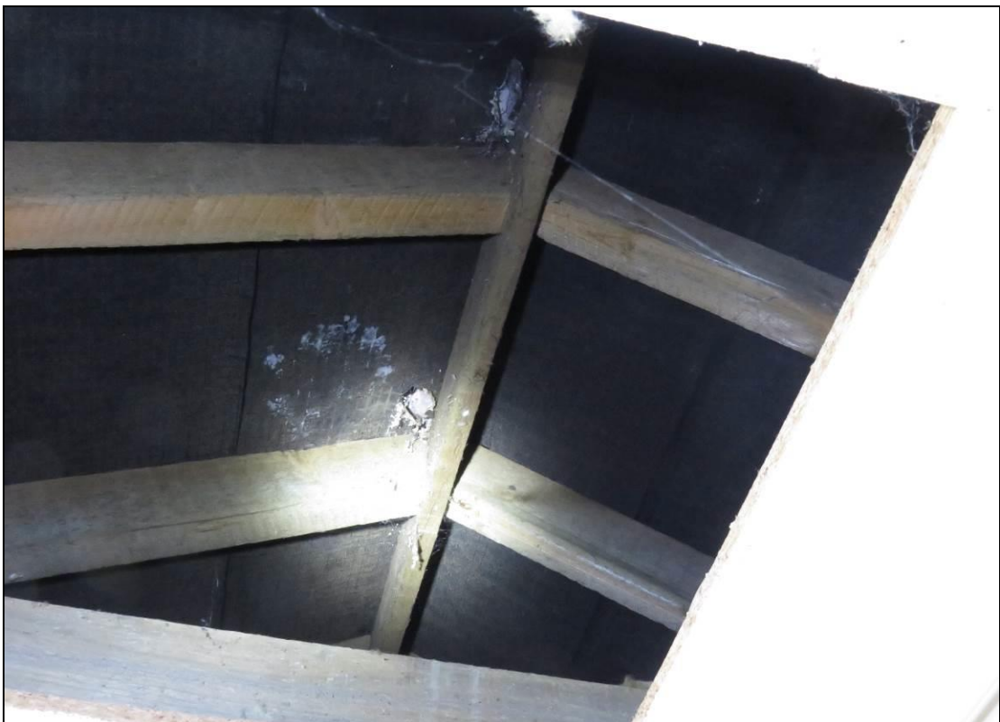
Photo 11: Loft Void of garage from Internal Inspection – no evidence of bats recorded , upper loft void with cobwebs indicated no recent use
