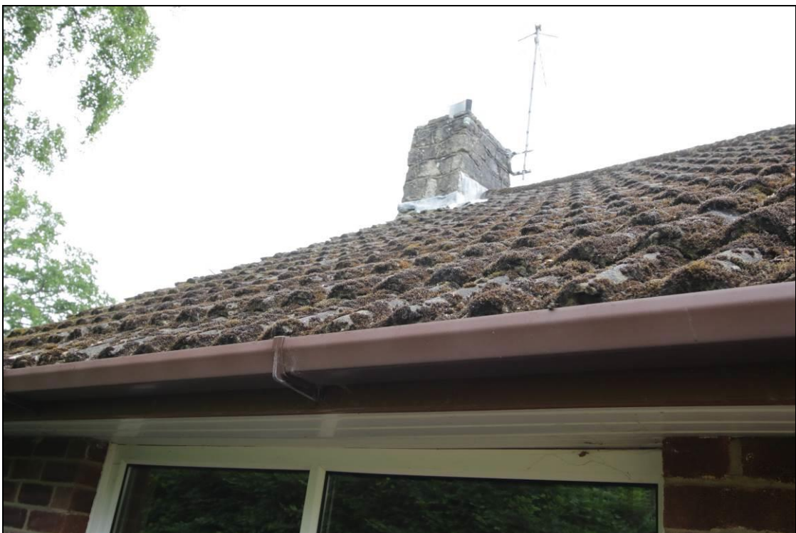
Photo 3: Interlocking roof tiles, ridge tiles and soffits are generally well sealed with few gaps
