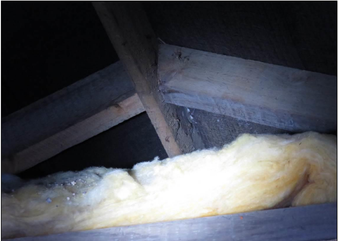
Photo 10: Loft Void of garage from Internal Inspection – no evidence of bats recorded , upper loft void with cobwebs indicated no recent use
