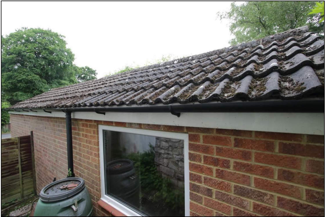
Photo 4: Single storey garage with interlocking roof tiles, ridge and soffits also mostly well sealed
