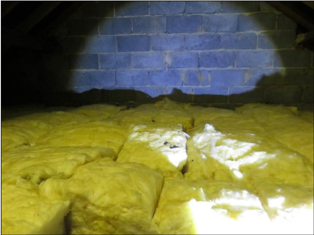
Photo 6: Loft Void from Internal Inspection – no evidence noted
