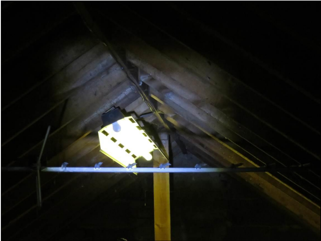
Photo 8: Loft Void from Internal Inspection – no evidence of bats recorded , upper loft void with cobwebs indicated no recent use
