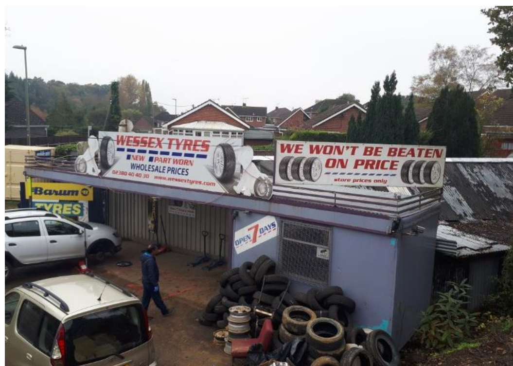
Figure 2 – Main Workshop Building (viewed from Providence Hill)
