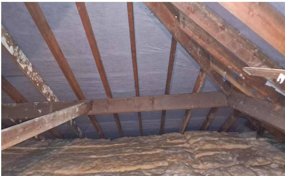
Picture 4: Showing the internal structure of the roof and the breather membrane.
