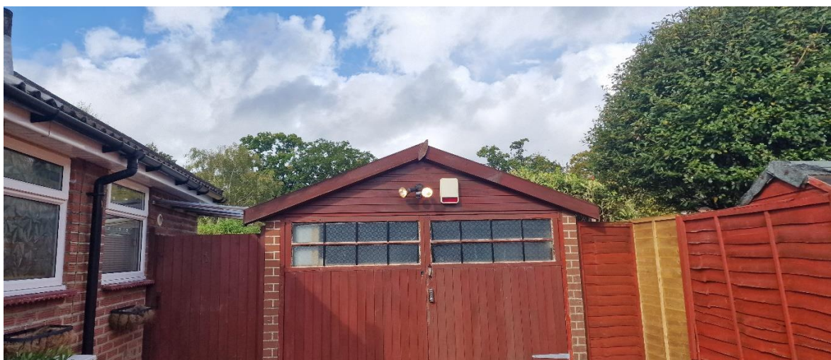
Picture 3: Showing the garage building.
