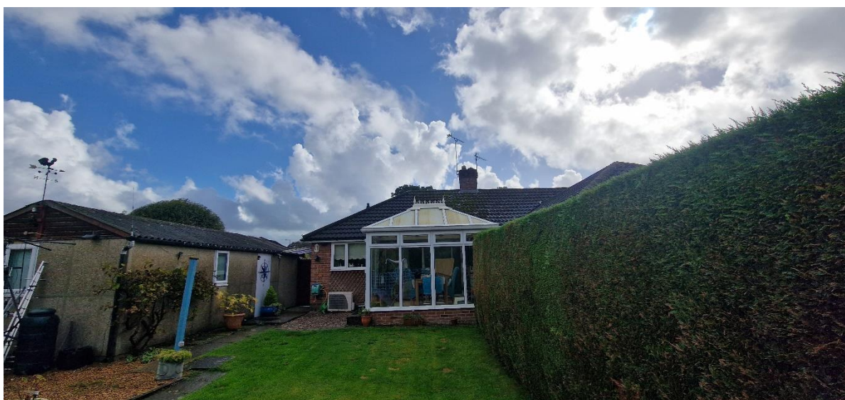
Picture 2: Showing the rear elevation and the garage building
