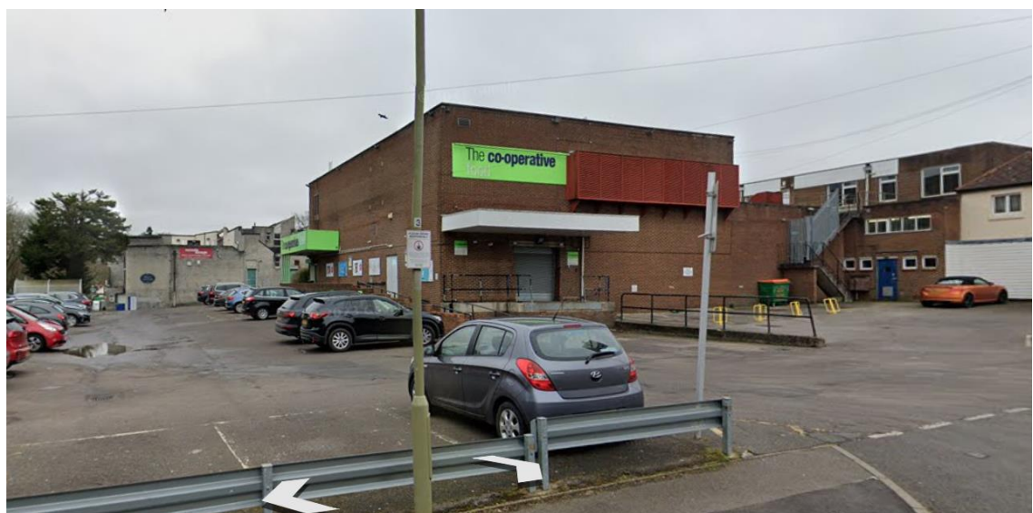
Figure 2 – Rear element of building – the application site
