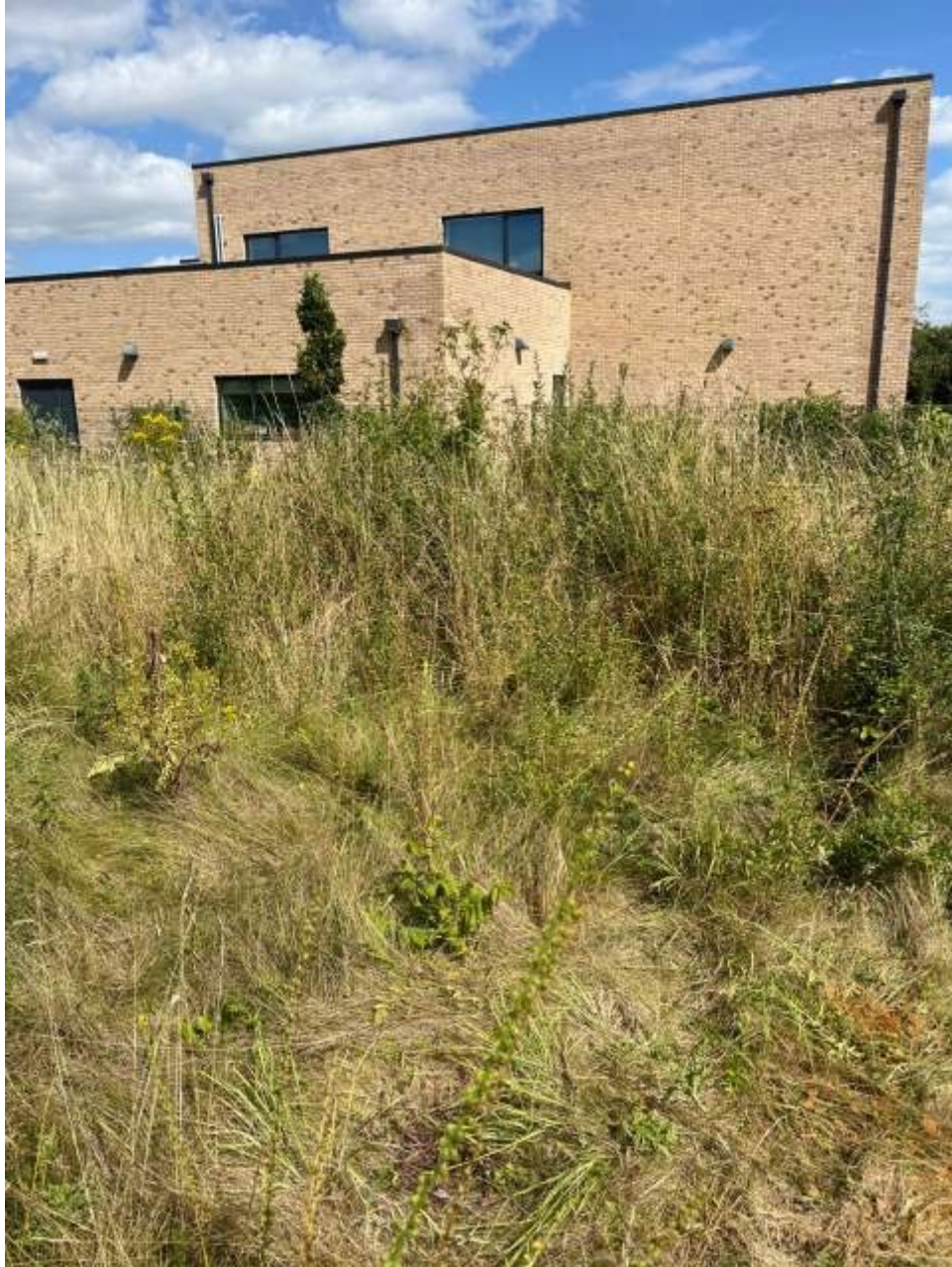
Plate 10 – A small overgrown stockpile east of site with school visible in background.
