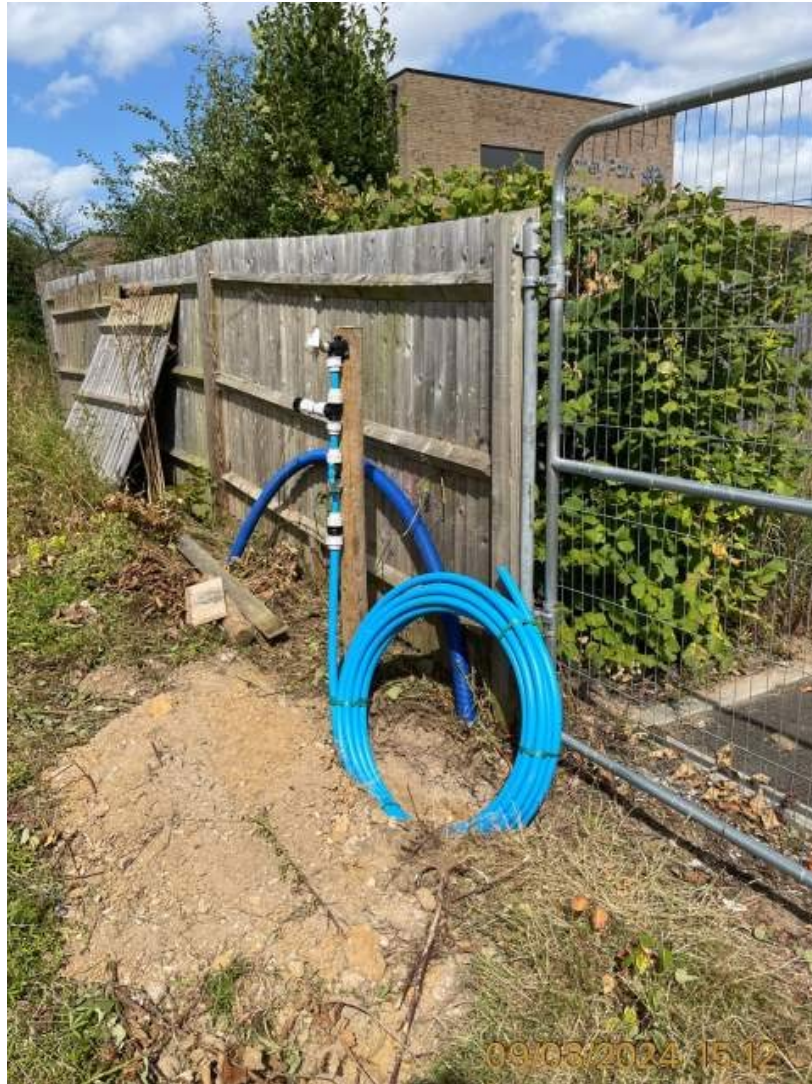
Plate 12 – A tap and pipework being installed on the day of site visit located at the site entrance.
