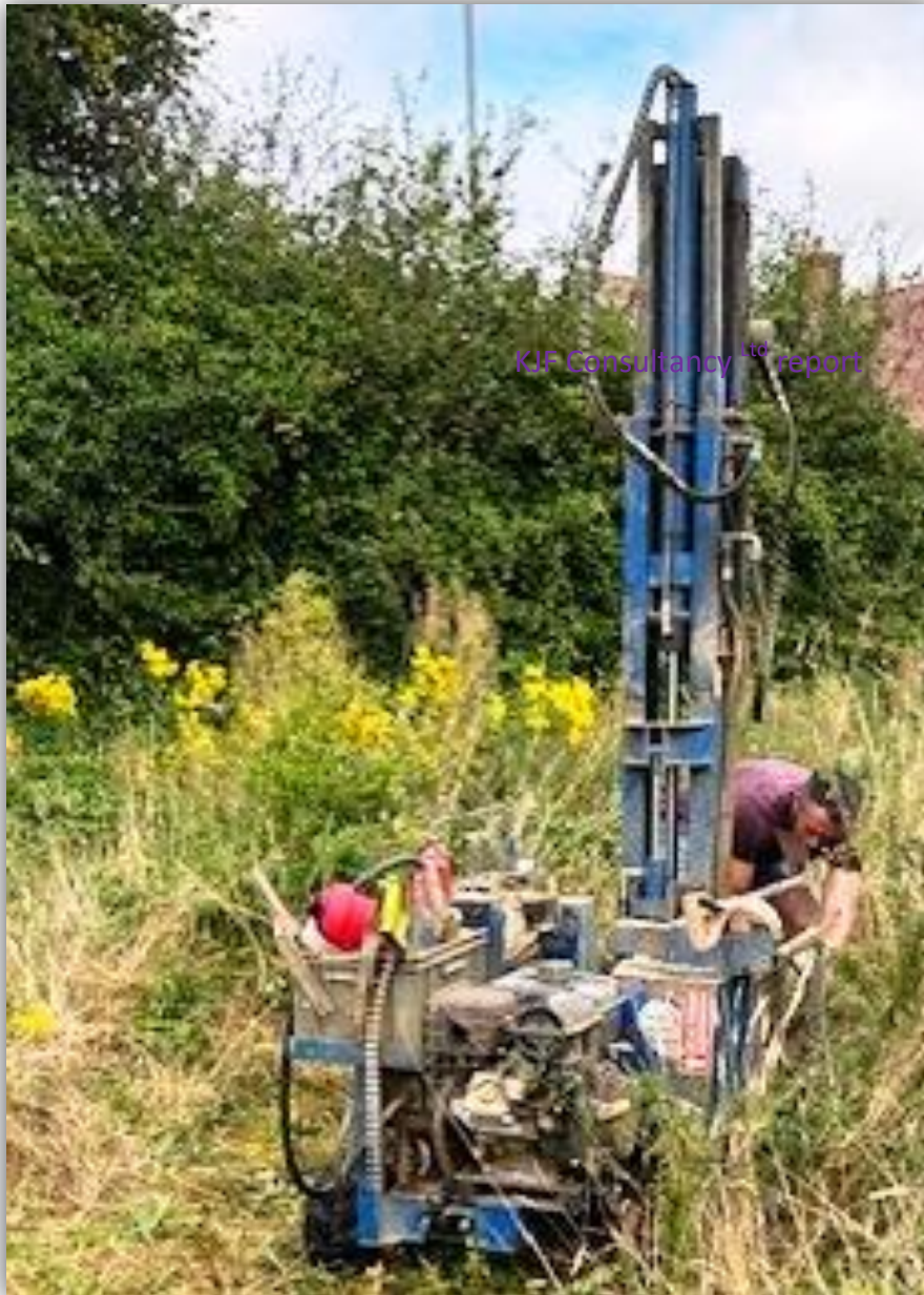
Small tracked rig used to extract soil from the boreholes.
