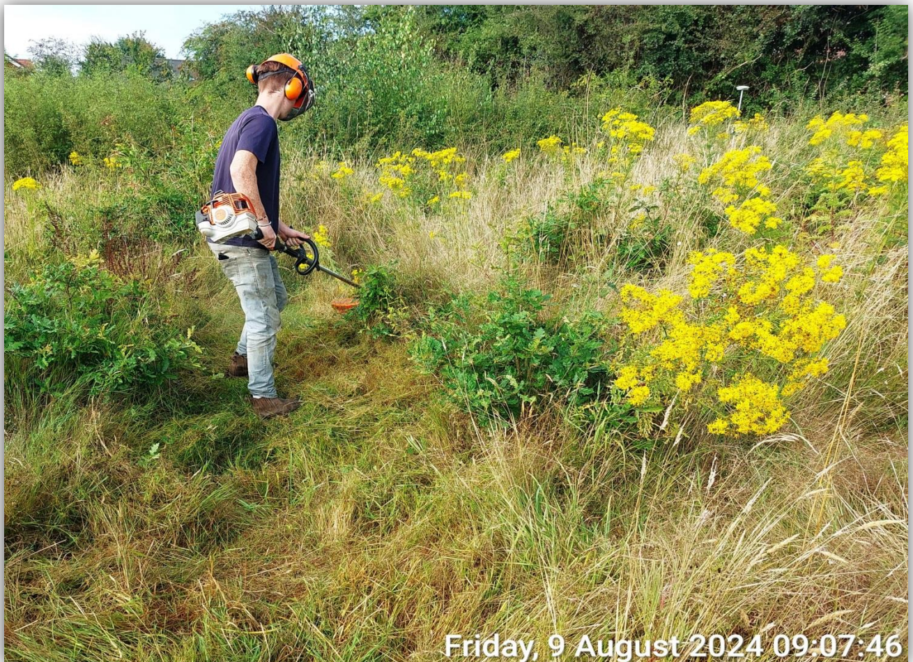
Strimmer used to make paths to the borehole locations.
