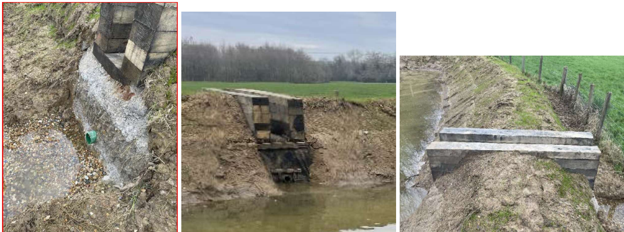
Photos included on As Built Survey.
