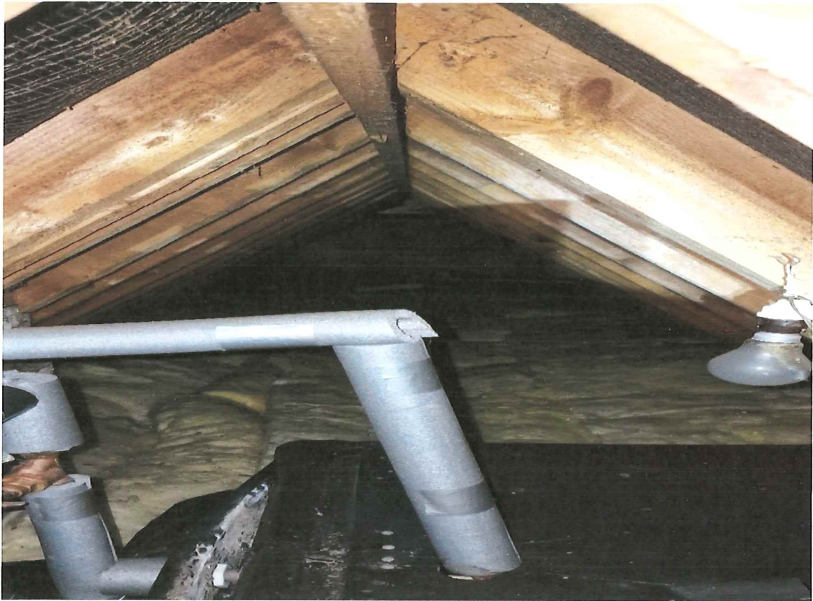
Picture 5: Showing the internal structure of the building and the thick layer of insulation.
