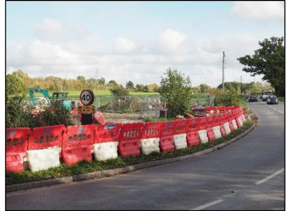
Photo 14 Defunct remnant hedgerow at A3351/A334 junction.
