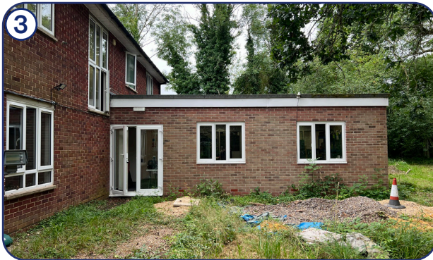
North west elevation of the existing buildings from the rear gardens looking south east
