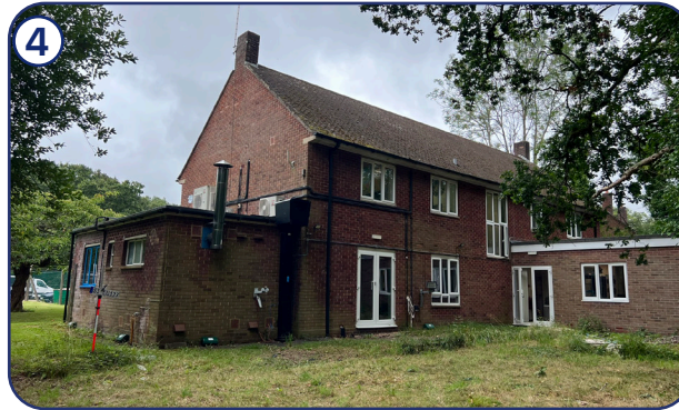
View of the existing building looking east
