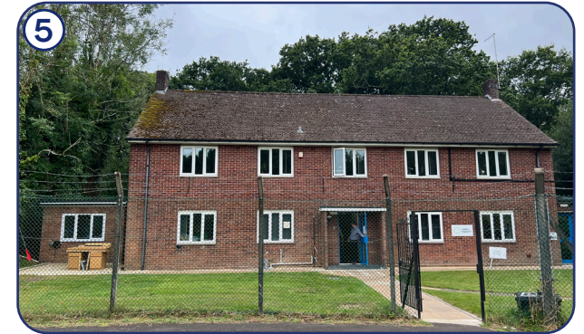
North east elevation of the existing building from the front lawn looking south west
