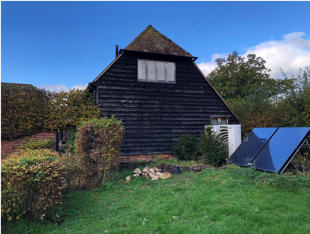
PHOTO 1: VIEW OF EXISTING EAST WALL OF NORTH BARN SHOWING HEAT PUMPS AND SOLAR PANELS
