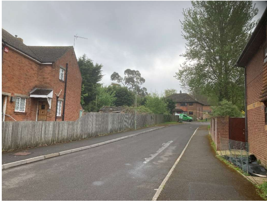
Fig. 2 – Photo taken on the corner of Kinsbourne Way looking south-east along Kinsbourne Rise (14 Kinsbourne Way on left).
