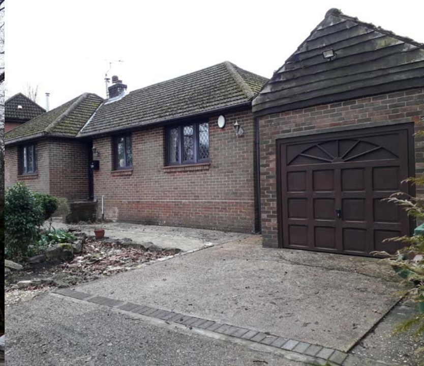
Existing Garage from Front
