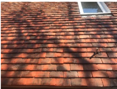
South western side of the house where the proposed extension will join to the existing house. A small triangle of hanging tiles will need to be removed and a small area of roof tiles on the garage will be disturbed to facilitate the construction of the new extension
