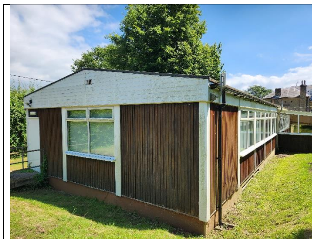
Photograph 19: The Annexe, viewed from the northwest.
