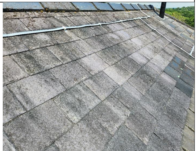
Photograph 14: Tightly fitting slate tiles across most of the roof.
