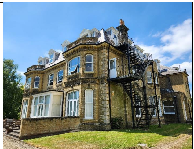
Photograph 12: The Main House, viewed from the east.
