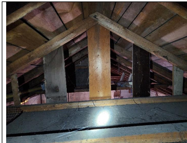
Photograph 27: The partially enclosed loft void at the northern end of the Barn.
