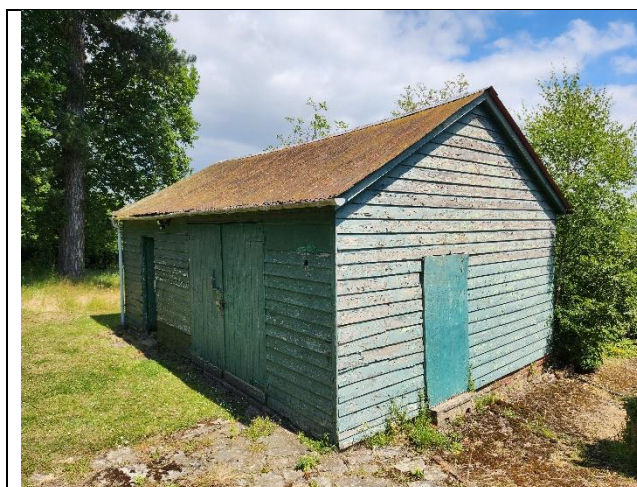
Photograph 23: The Barn, viewed from the southwest.
