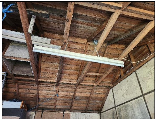
Photograph 28: The southern end of the Barn, open to the rafters.
