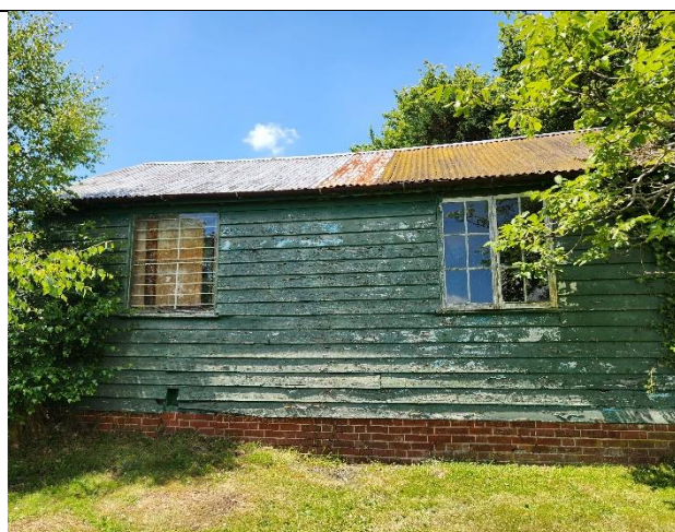
Photograph 24: The Barn, viewed from the east.
