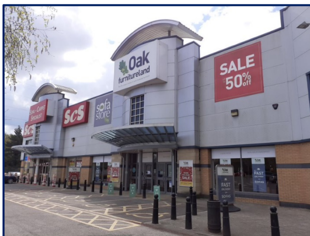
Photograph 5: Offsite industrial unit connected to onsite building.
