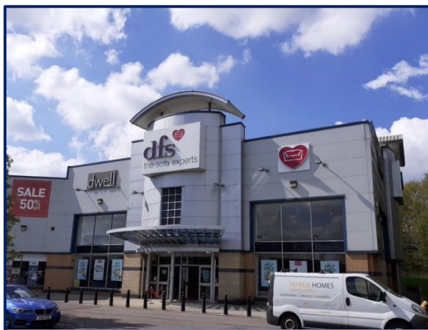
Photograph 1: Current DFS store onsite.
