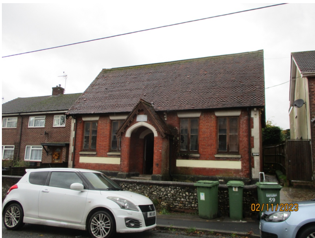
View of the front elevation.
