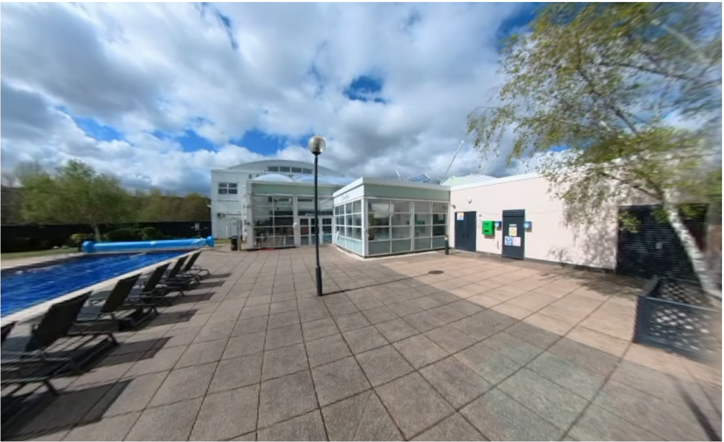
Photo 2 Proposed Spa Extension & Garden Location Photo
