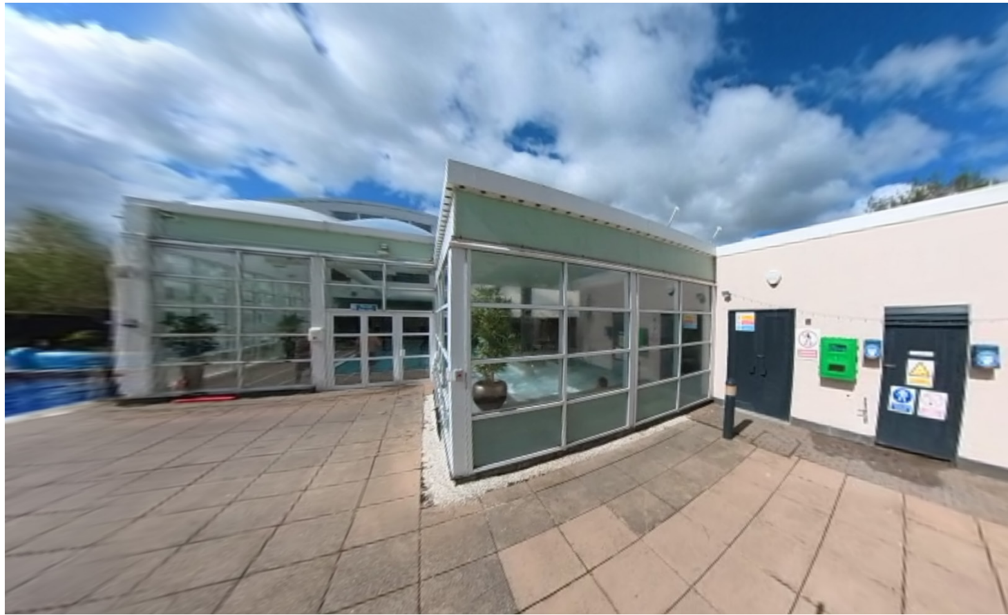
Photo 1 Existing Part Of Spa To Be Extended
