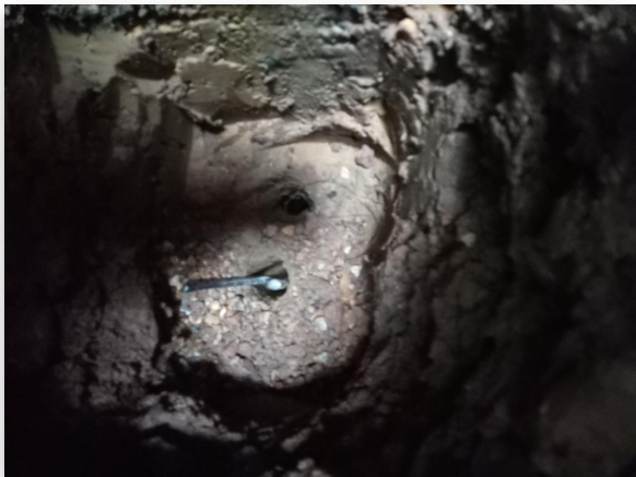
Fig 1.2: Trial Hole 1 Footing
