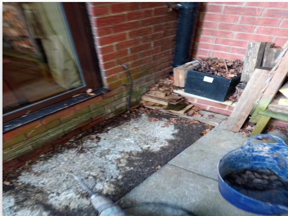
Fig 1.1: Trial Hole 1 Location
