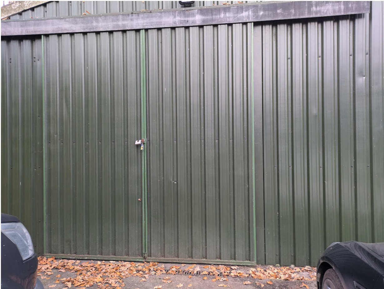
Figure 5.1 – Main doors to building
