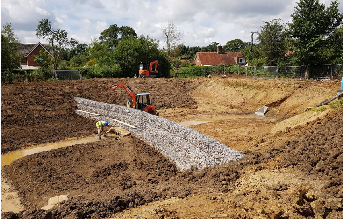
Detention Basin During Construction – View south
