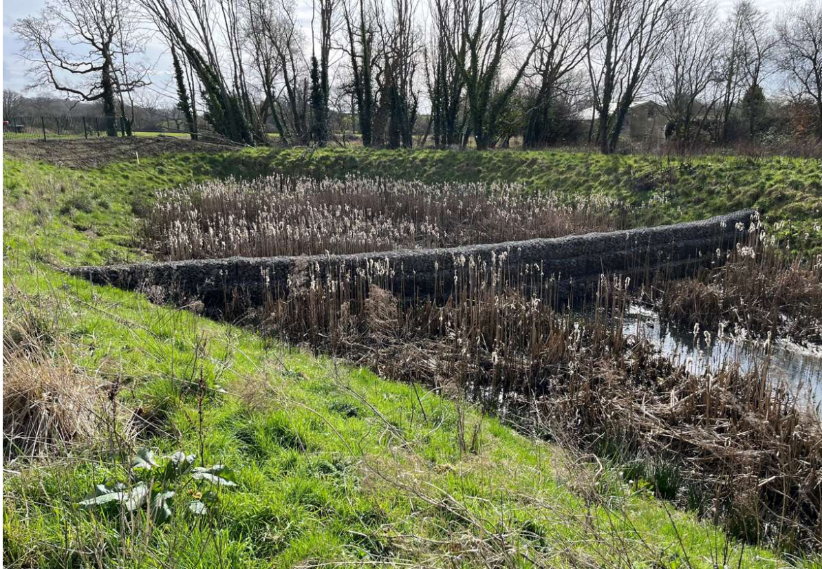
Completed attenuation – View east
