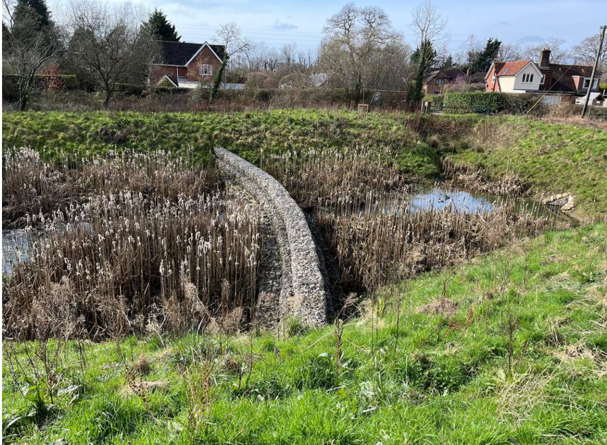
Completed attenuation – View south
