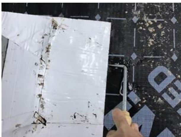
Pick testing all SAGM detailing.
