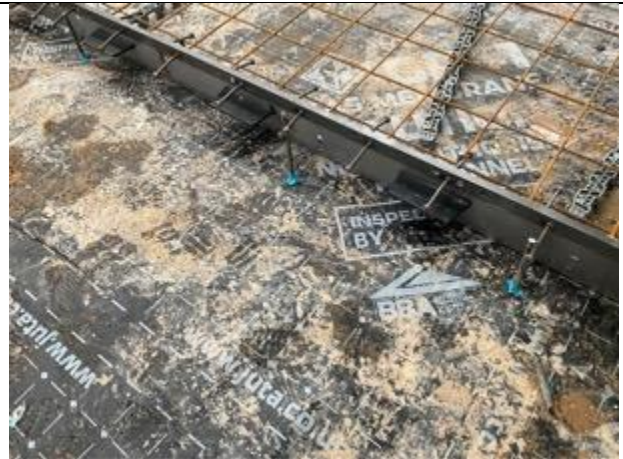
Armoured joint pin's left in and a continuous band of double sided butyl tape wrapped around.
