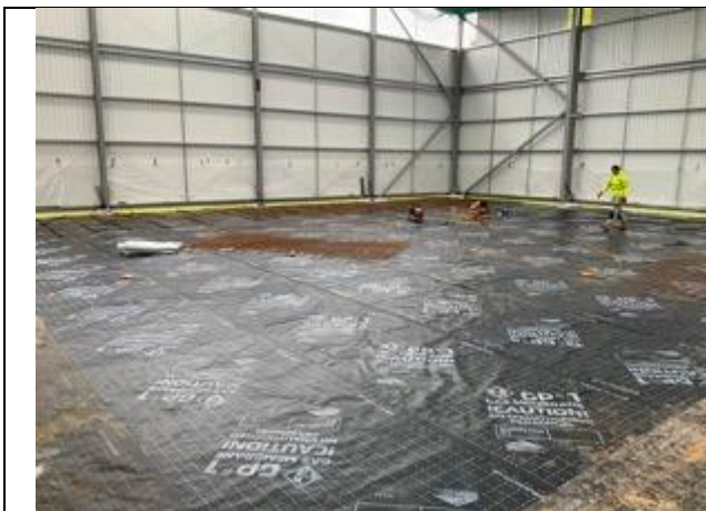
Overview of the full footprint installation of Juta GP1 Gas Barrier.
