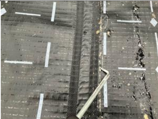
Pick test upon a auto welded membrane lap joint.
