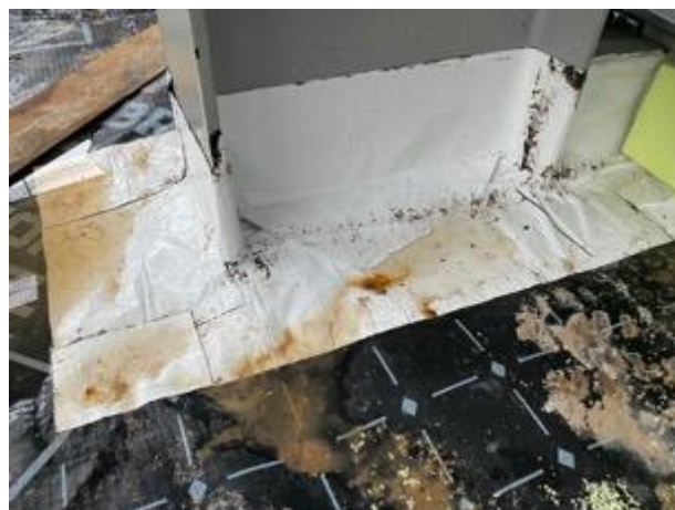
Typical steel stanchion sealed using SAGM
