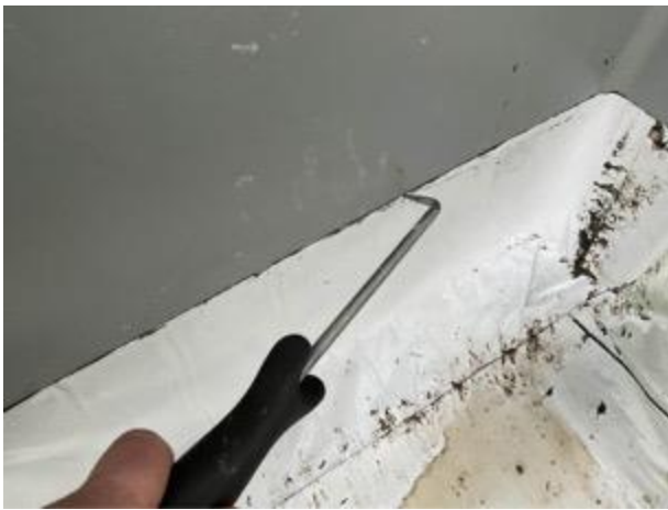
Pick test upon a sealed steel stanchion.
