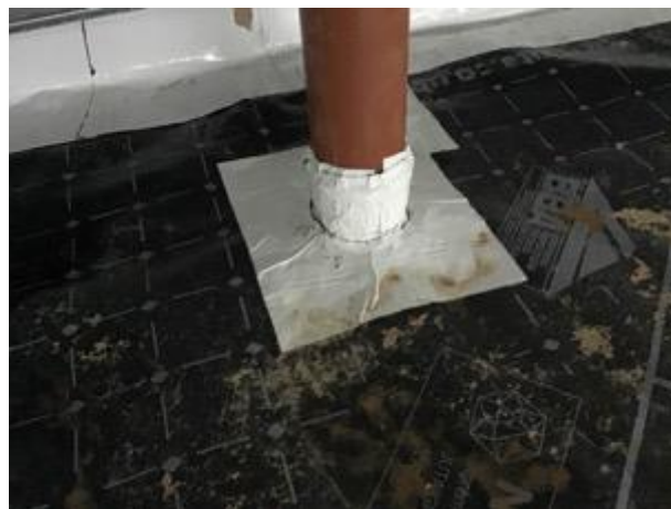
Typical pipe penetration seal using SAGM.
