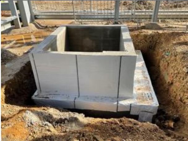
Unit 3/4. Overview of Lit pit wrap installation.
