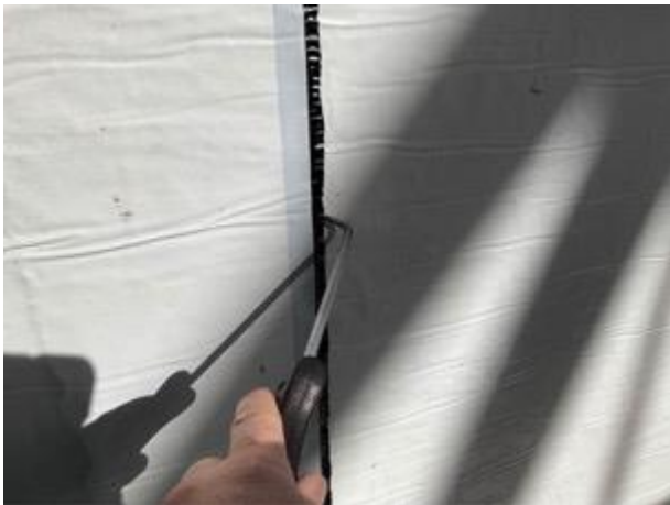
Unit 3/4. Pick test conducted membrane lap joint.
