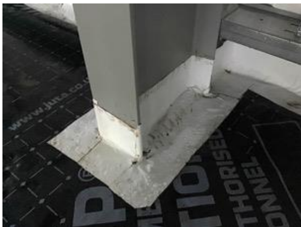
Typical stanchion seal using SAGM.
