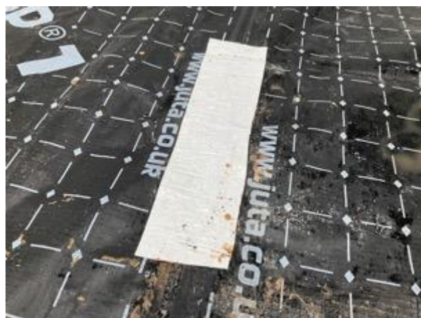
Patch repair using SAGM.
