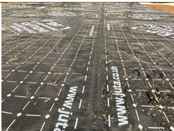
Auto welded membrane lap joint.
