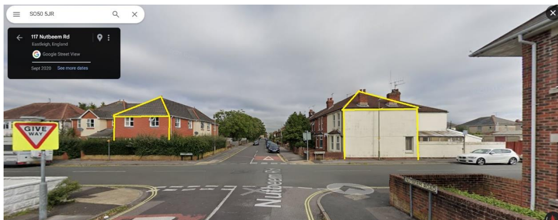
Figure 1. Photo section of Nutbeem Road, highlighting with yellow the existing character/shape of the blocks
