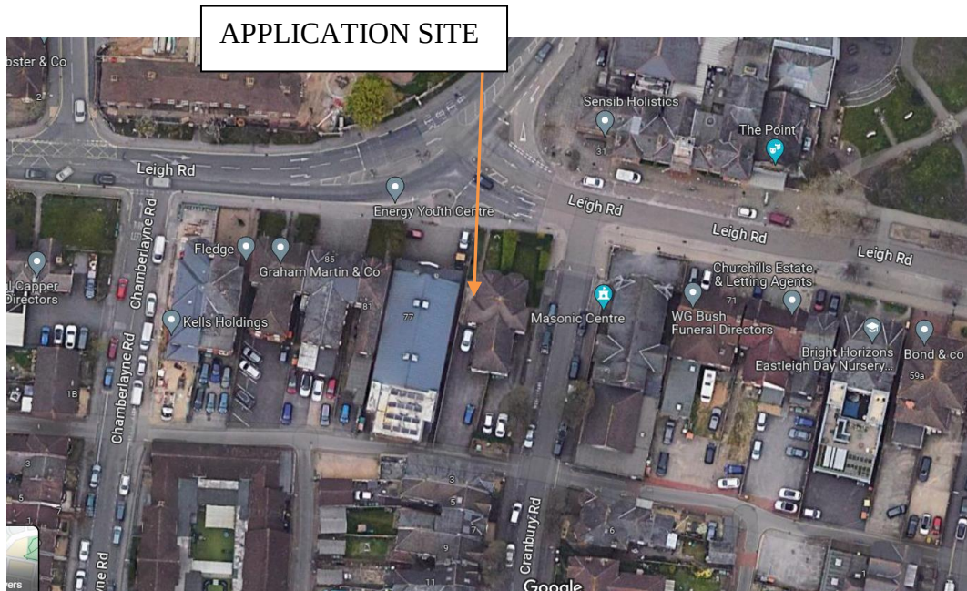
Aerial Photo showing No 77 Leigh Road (courtesy of Google maps)
