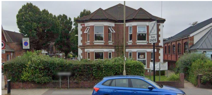
Photo 1 – the existing hedge in front of Nos 75 and 77 Leigh Road
