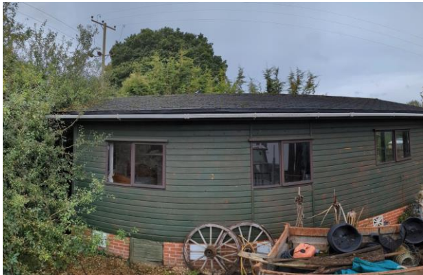
Figure 4: B1 viewed from the east.
