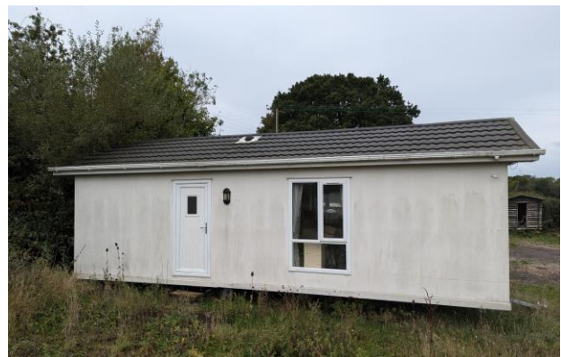
Figure 9: B2 viewed from the east.
