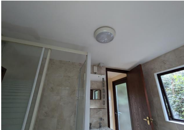
Figure 6: B1 internal space, ceiling.
