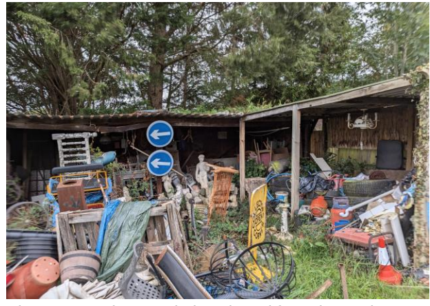
Figure 13: B4 lean to shelter viewed from the north-west.
