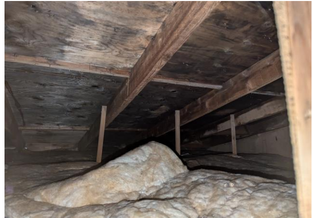
Figure 7: B1 roofspace with insulation.
