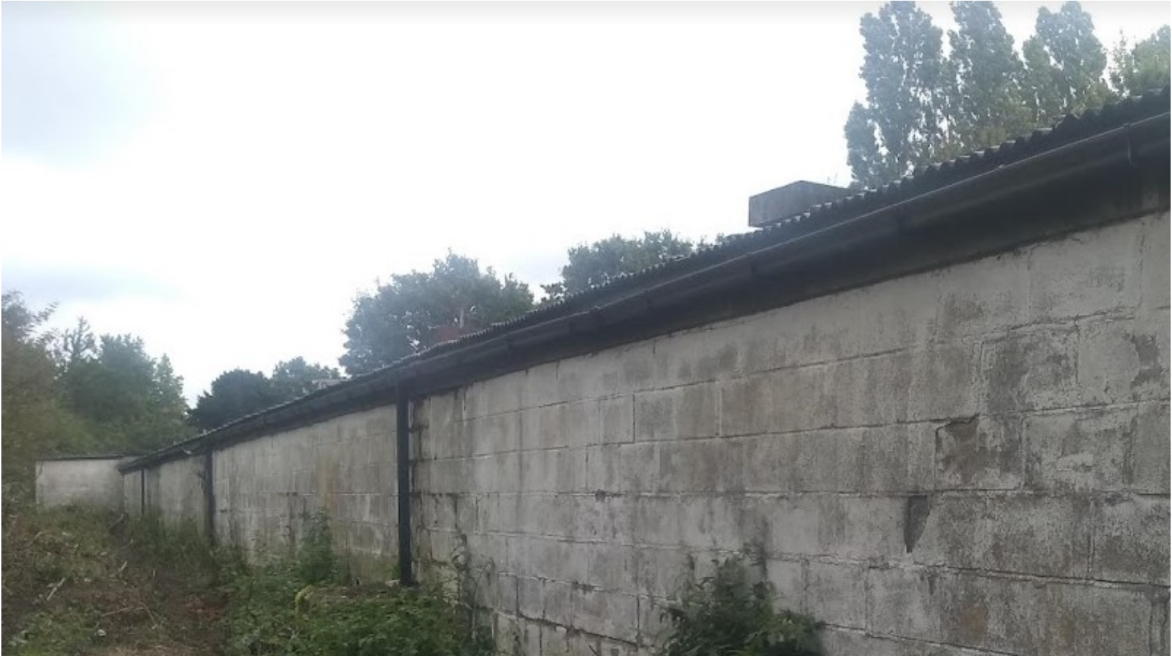
External blockwork walls
