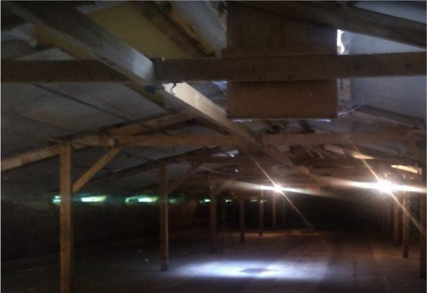
Internal roof timber roof support frames
