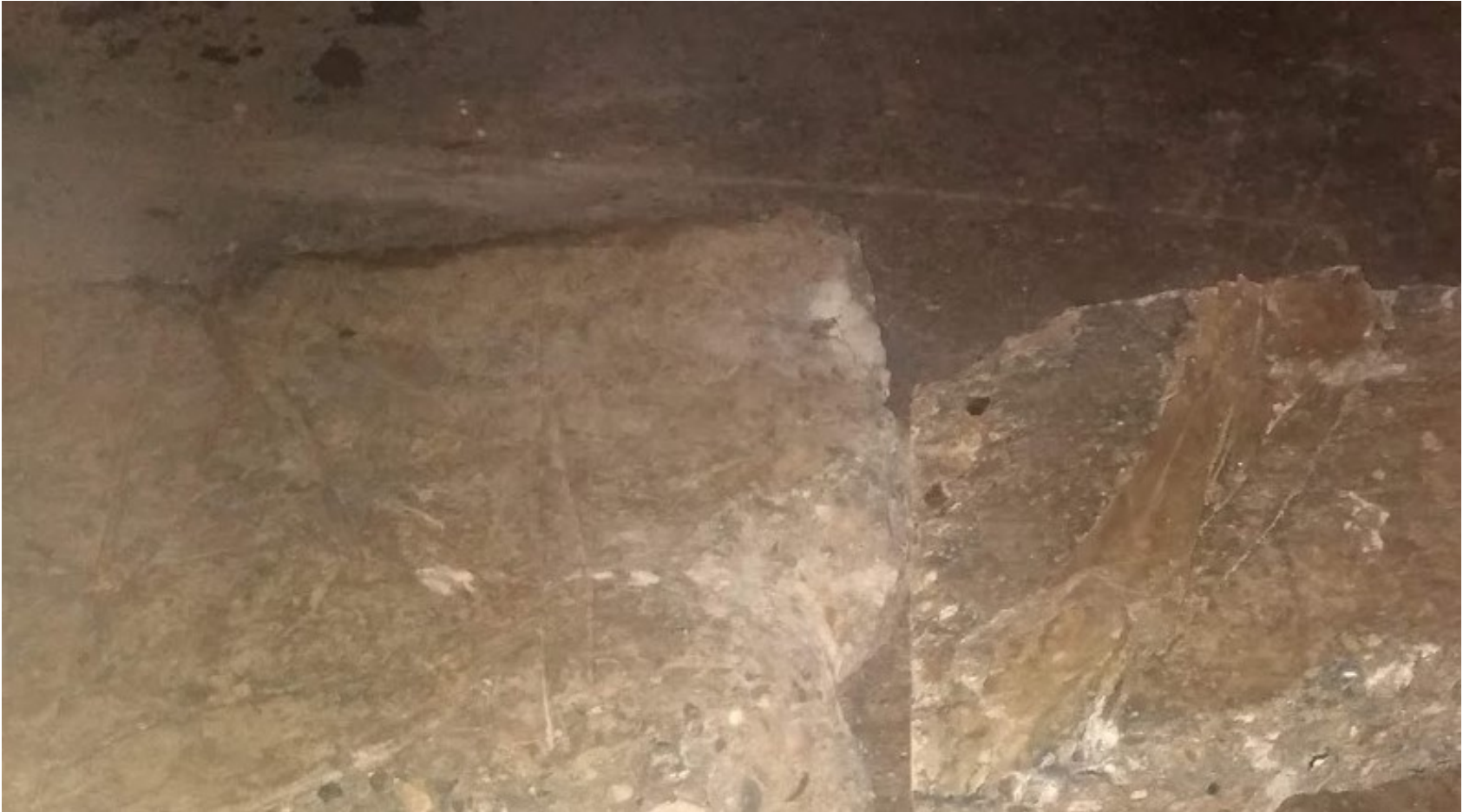
Concrete ground floor slab revealed in trial hole
