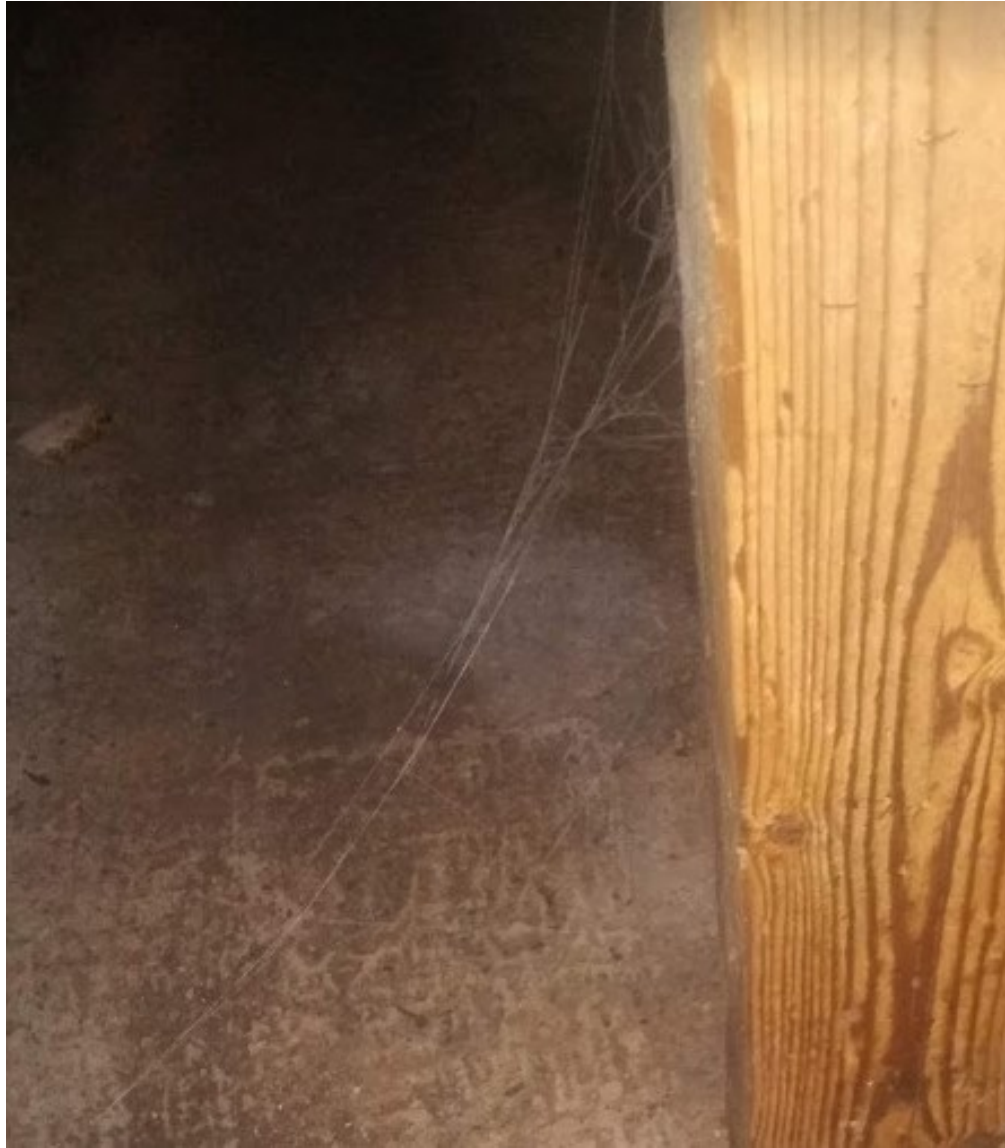
Structural timber support posts supported on ground floor slab
