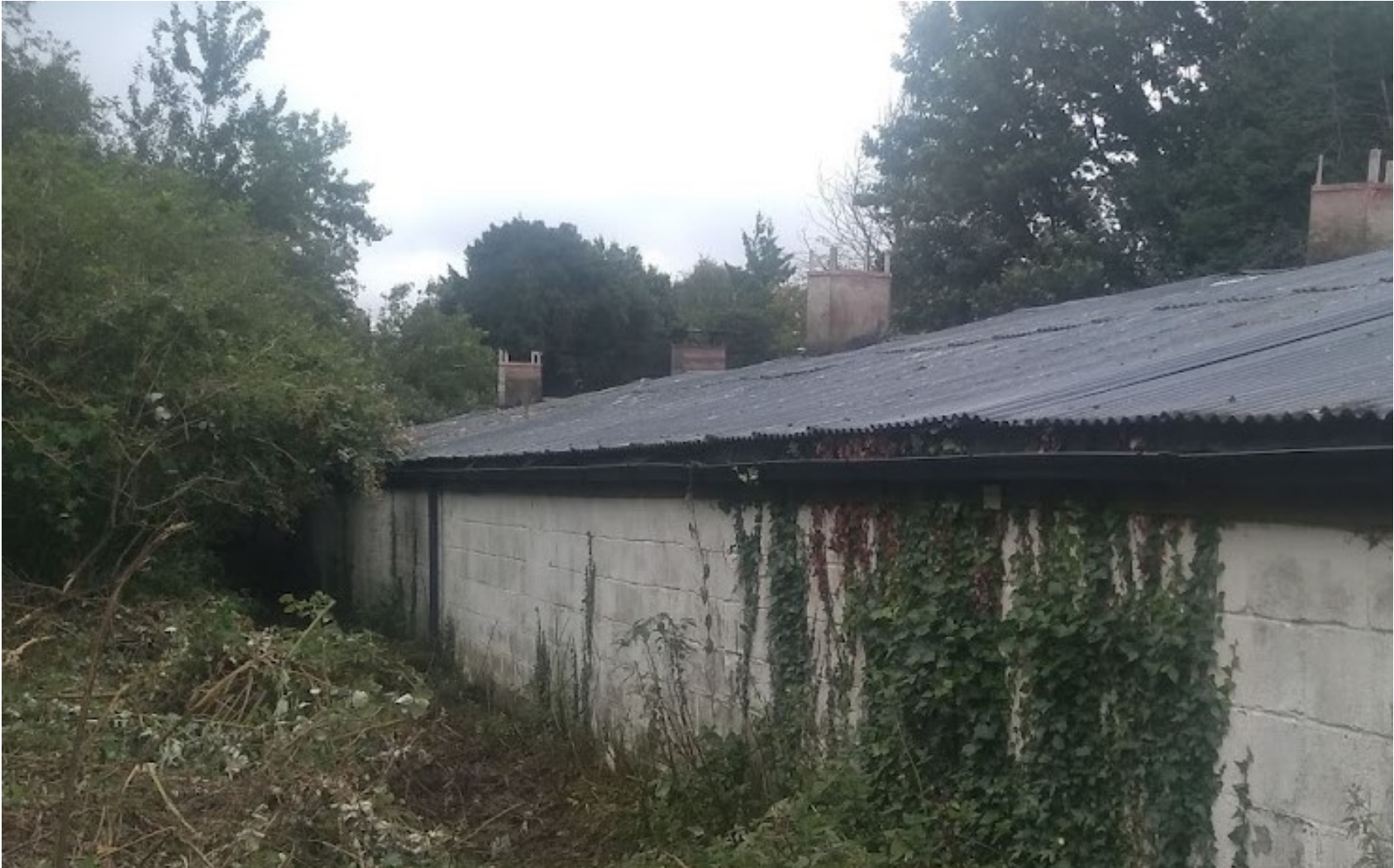
External blockwork walls with metal sheet roofing
