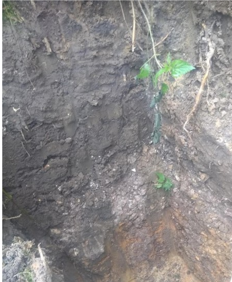
Concrete foundations revealed in tril hole
