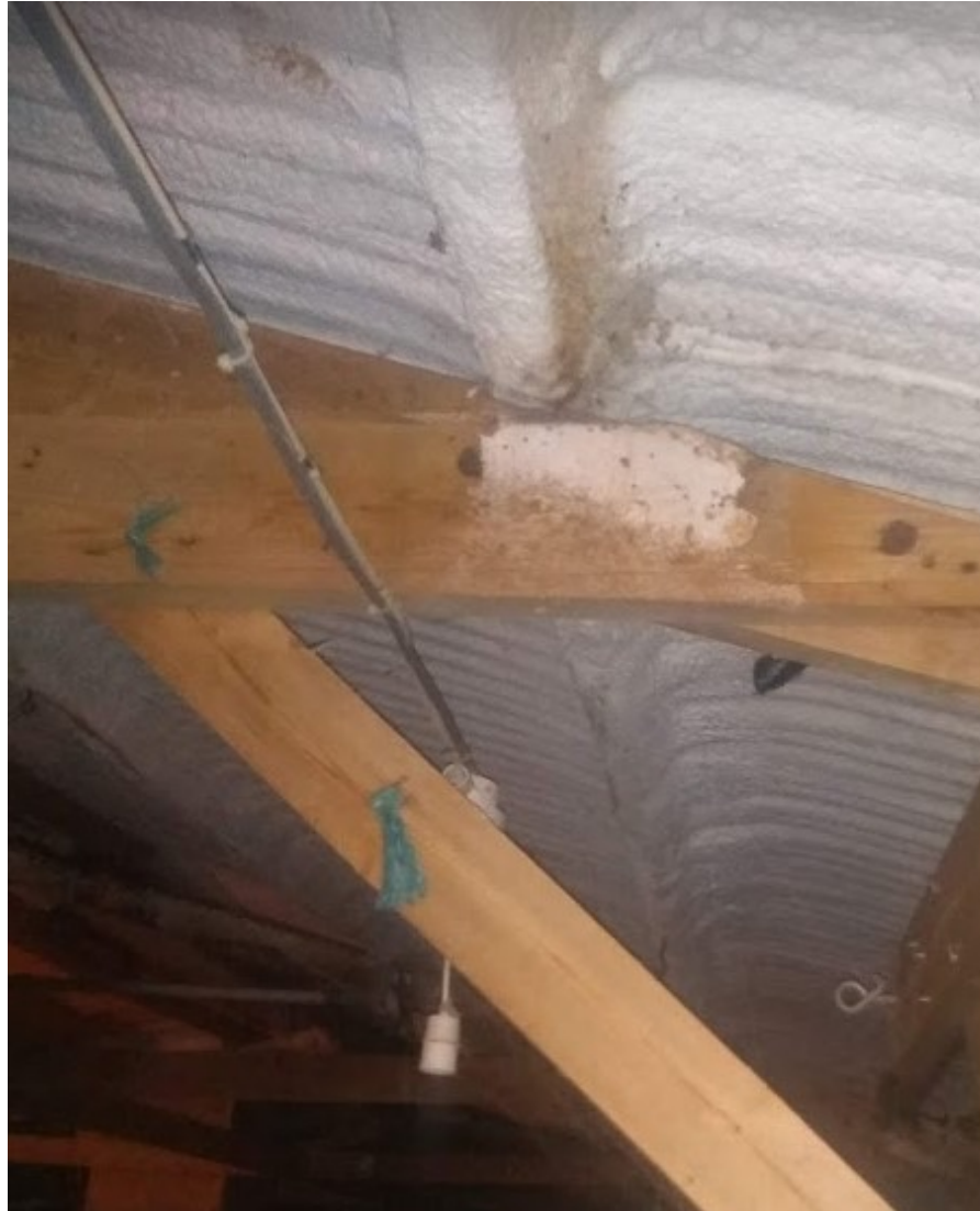
Internal roof timber roof support frames
