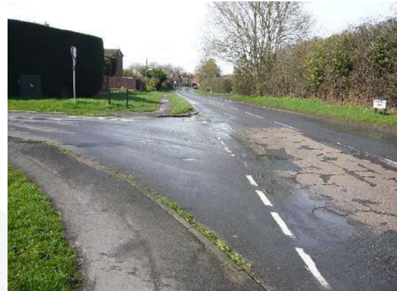
View north along Winchester Road
