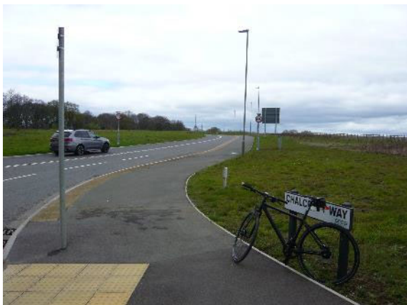
Shared facility on Chalcroft Way
