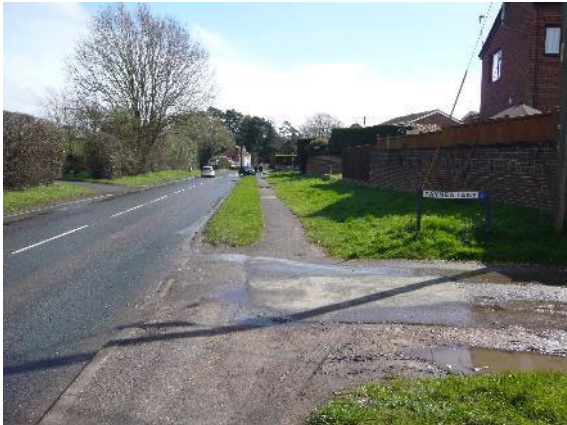
View south along Winchester Road
