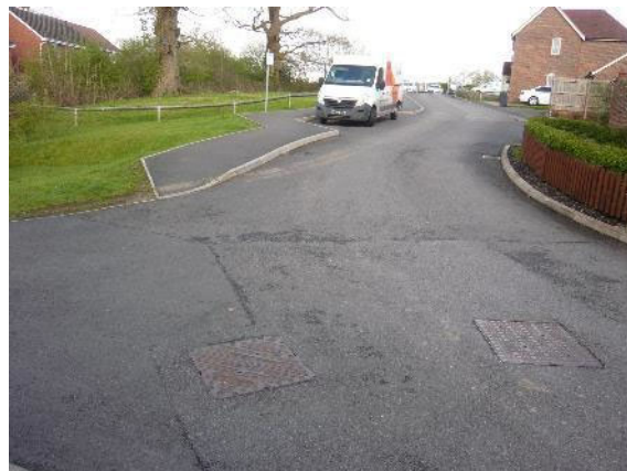
View along Knowle Park Lane
