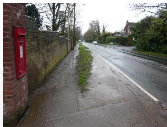
View south-east along Mortimers Lane (north-east of Mimosa Drive)
