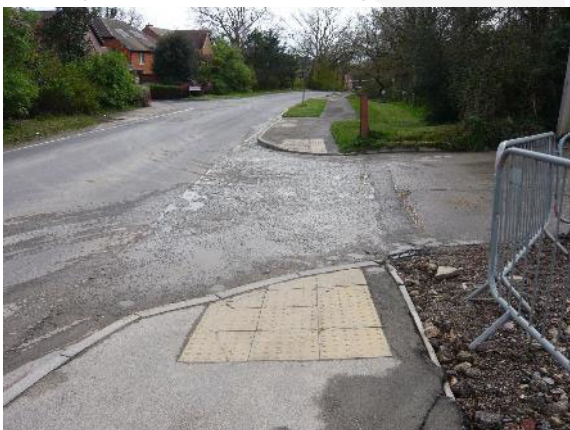
View along Knowle Lane
