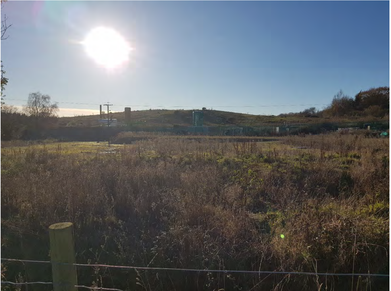
Plate 17 View of the offsite Fair Oak Landfill with gas extraction system
